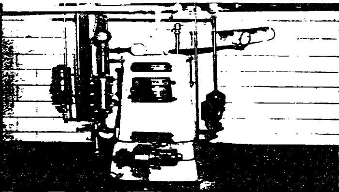
Fig. 13—Water Tank and Boiler Domestic Fuel Oil Burner Insulated With INSULAG.
