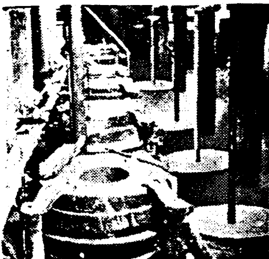
In 1899, the old Calumet factory equipment was removed and replaced with twelve 30-inch standard S-W liquid paint mills, mixers, and thinning tanks. The chief products were SWP, floor enamel, and roof paints.
