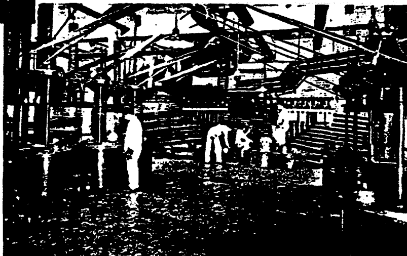
Building No. 23 was erected in 1921 to provide additional equipment for the manufacture of high quality enamels and other liquid paints. The equipment included 15 tandem mills, 4 roller mills, 38 mixers, and 38 thinning tanks. The daily capacity was 4,000 gallons.
