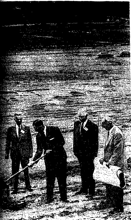
E. Loiseau, president of Public Service Co., breaks ground for the Cherokee power plant to be built by the company at E. 62d and Franklin St. With him are M. M. Koch (left), vice president; LeRoy R. Patterson (second from right), assistant vice president, and Ben Snow, contractor.
