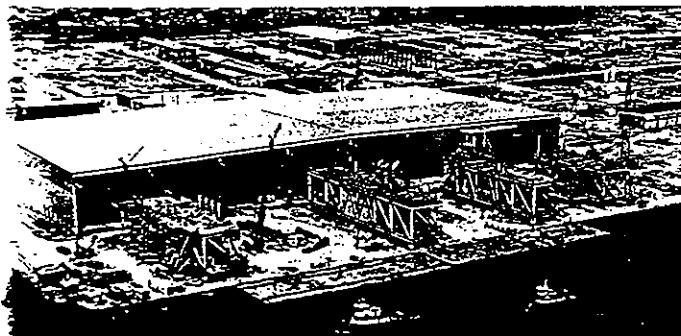
Deck modules for the Mars TLP, JRM's second TLP project for Shell, were completed at the Morgan City, Louisiana fabrication yard. Modules for Shell's next TLP are now under construction at the yard.
