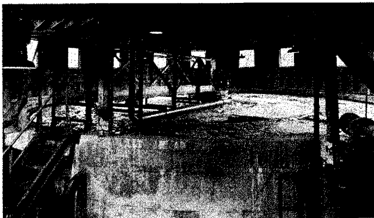
THICKENER RECOVERING FINE RUBBER STOCK AT THE RUBBER RECLAIMING PLANT OF THE GOODYEAR TIRE & RUBBER COMPANY AT AKRON
