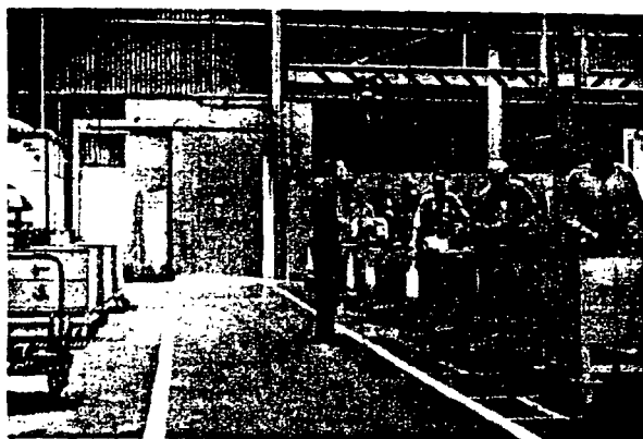
The electrical shop in Central Shops is one of the areas where outstanding housekeeping makes the area exceptionally neat and safe. The Central Shops area has received high scores during inspections under the new Special Emphasis housekeeping program.
