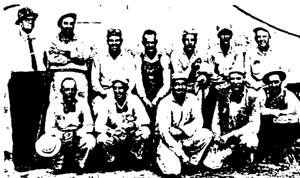
Among those assigned to the No. 30 TEL storage tank dismantling job were, front row, left to right, Sid Cowart, Operations foreman; Ralph Simmons, ironworker 1/c; George Kelly, rigger 1/c; Charles A. Bozeman, rigger helper 1/c; and F. E. Doughty, rigger 1/c. Back row, left to right, E. J. Lorio, area safety engineer; Mike Jeansonne, Construction foreman; Branch Goux, welder 1/c; Henry L. Harless, welder 1/c; Ewell Melancon, ironworker 1/c; Edward Y. Easterly, rigger 1/c, and R. L. Blackledge, rigger 1/c.
