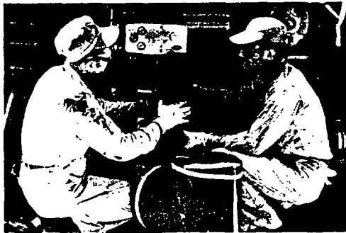
B. E. Duplessie, left, insulator 1/c, and W. W. Harris, insulator helper 1/c, are shown performing a construction function. They are installing insulation on a propane control station. Construction workers in all Plant areas improve existing equipment or build new facilities.
