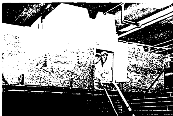
Entry into the "Smithmobile" is through a door at left end, not shown. The hood at the top keeps falling scale inside the box and the doorway is for equipment hoses from below. In the door are L. J. Dugas and F. M. Hagler.
