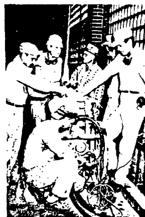
The crew working with the "Smithmobile" included, from left, Sam Accardo, E. A. Wascom, foreman, Robert Smith, supervisor, F. M. Hagler, B. B. Pate and L. J. Dugas, kneeling. Sam Butler also worked on the job but was not present when this picture was taken.
