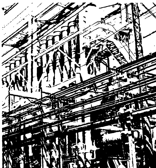
This jet refrigeration unit, one of the largest in the world, is another installation which cools water for further use after it has been used to reduce temperatures in the manufacturing processes. This installation is another expensive unit which conserves the water supply of the community.
