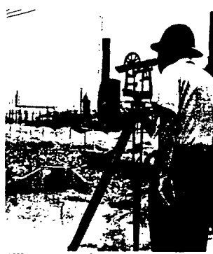
Bill Egan, civil engineer, checks the elevation and layout of the new culvert installation near the No. 2 Sodium Cell Room.
