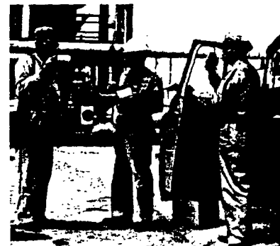
When "trouble" call is received from Bridges at Main Gate, Al Cotten, Security, demonstrates how patrol truck is rushed to scene with portable radio and megaphone for communications in problem area. Shown with Cotten are Fred C. O'Rourke, Operations foreman, and Percy Breeden, EtCl general foreman.
