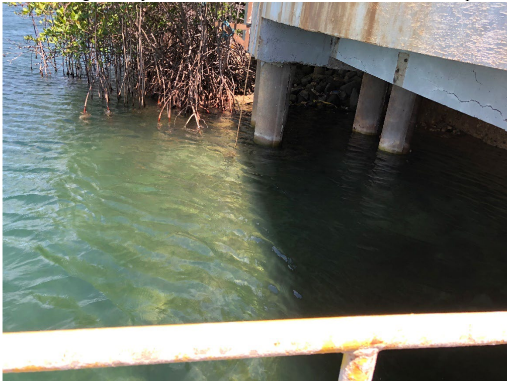
Photo #4. An on-site grab sample was collected from the intake structure for temperature.
