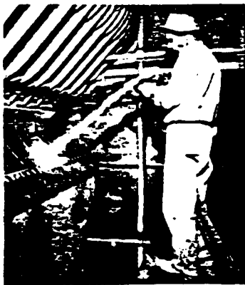
Cement gun applicator shooting R & I Moldit-D in place in ash hopper of large public utility boiler.
