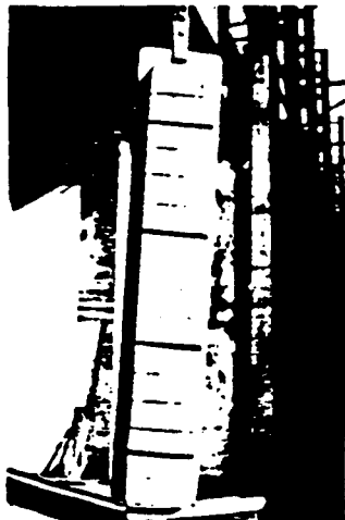
Moldit-A used to line these coke oven stand-pipes—still in good service after 18 years.
