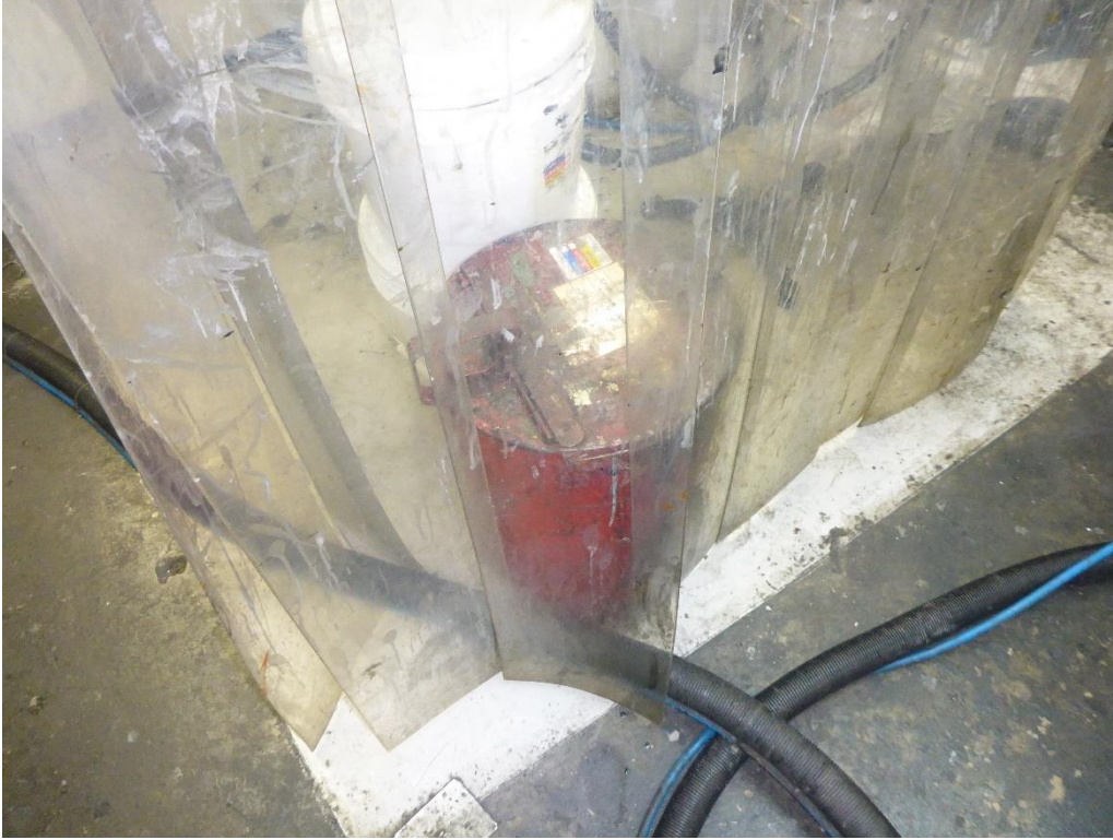
Photo 4: One flip-top 5-gallon container for accumulating solvent contaminated wipes in the Screen Print Area One. The container, which was located next to one of the roll coat stations, was not labeled “excluded solvent contaminated wipes.”
