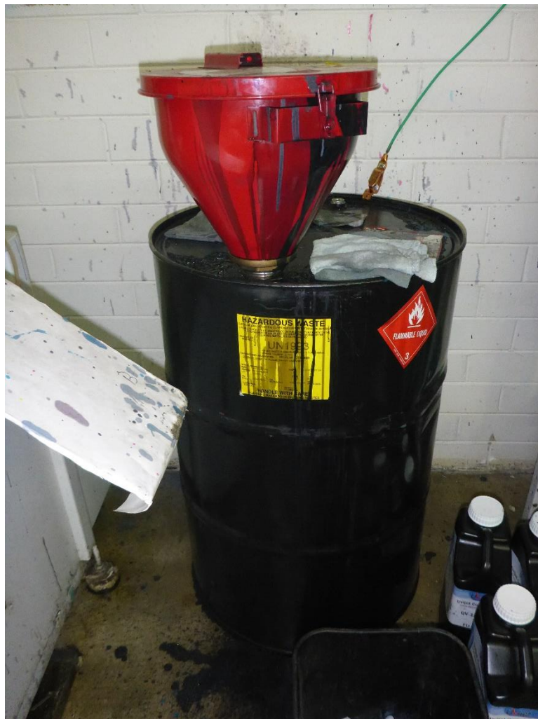
Photo 15: One 55-gallon container for accumulating hazardous waste in the lithographic area. The drum was identified with a flammable liquid hazard placard. Ink waste drips and spills obscured part of the hazardous waste label, but the container appeared to be labeled as D001 / F003 / F005 hazardous waste ink sludge with UV component (mineral spirits).
