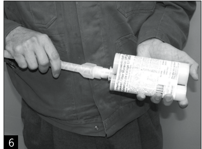
6 ... and screw on static mixer until it is firm. Connect compressed air to the air gun.
