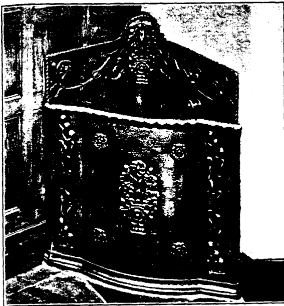
This detail of the handsome lead cistern in the Erickson residence should be of interest to architects and designers.
