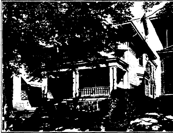
Pure white lead paint on this house outlasted a neighboring job with another paint by more than 2½ years.
