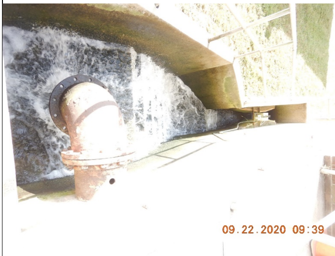
5: DSCN0041.JPG Location: Crane Naval Surface Warfare Center Photographer: Jonathan Moody Date/Time: 9/22/2020 9:39 AM Camera Direction: South Description: At the flume, downstream of the sand filters, where flow is monitored. Looking downstream at a step aeration system.
