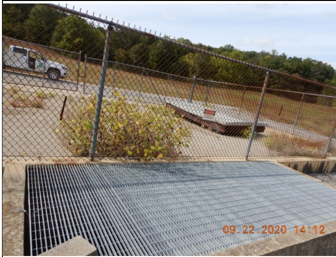
24: DSCN0060.JPG Location: Crane Naval Surface Warfare Center Photographer: Jonathan Moody Date/Time: 9/22/2020 2:12 PM Camera Direction: Northwest Description: Pit #1 and Pit #3 where ammunition boxes and treated wood are burned. Runoff from these sites flows into the blind sump under the grate in the foreground. Outfalls 016 and 017 are monitored when the sumps are emptied.
