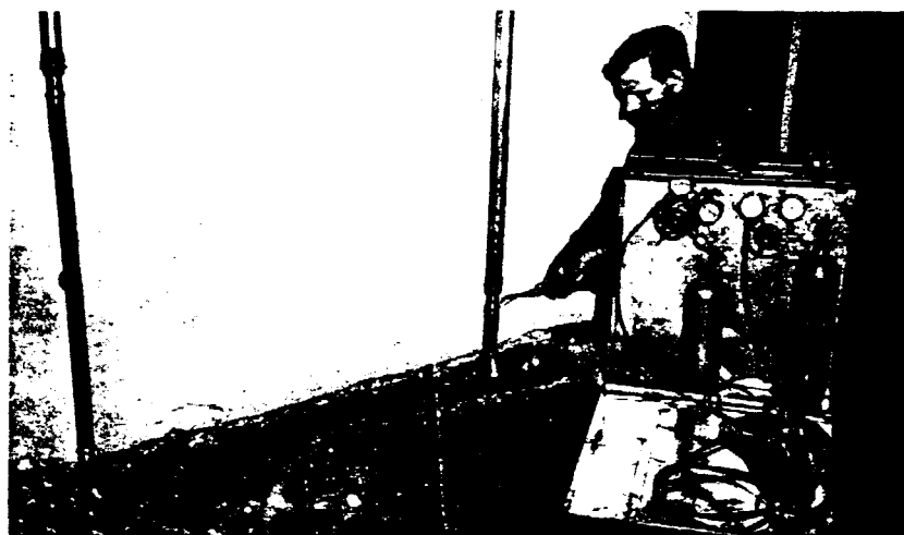
C. Vanzant, journeyman plumber of Denver, Colo., showing his ingenious portable lead welding kit in use in the field.
