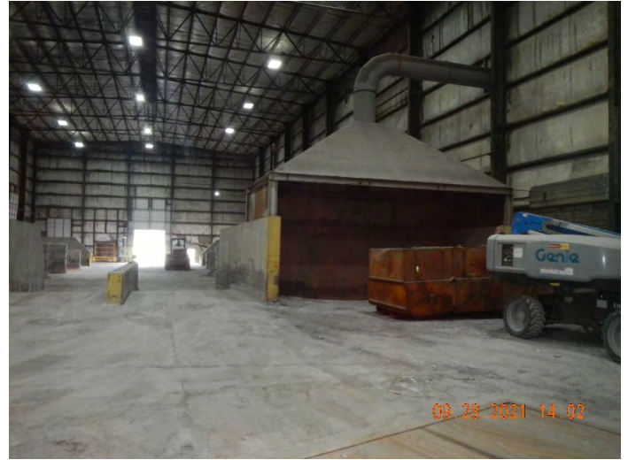
Photo #:14 (DSCN2519) Description: Facing north, photo of the salt cake storage/cooling area and associated capture hood near Rotary Furnace #6.
