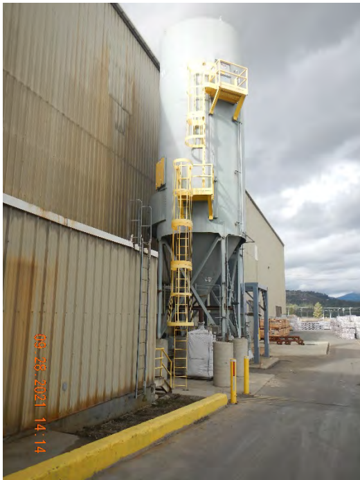
Photo #:15 (DSCN2524) Description: Facing north, photo of Baghouse #8. Used as a pollution control device for the salt cake staging and handling area near Rotary Furnace #6.
