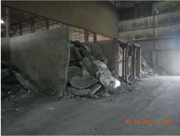
Photo #:13 (DSCN2506) Description: Facing southwest, photo of the dross storage area near Rotary Furnace #3.
