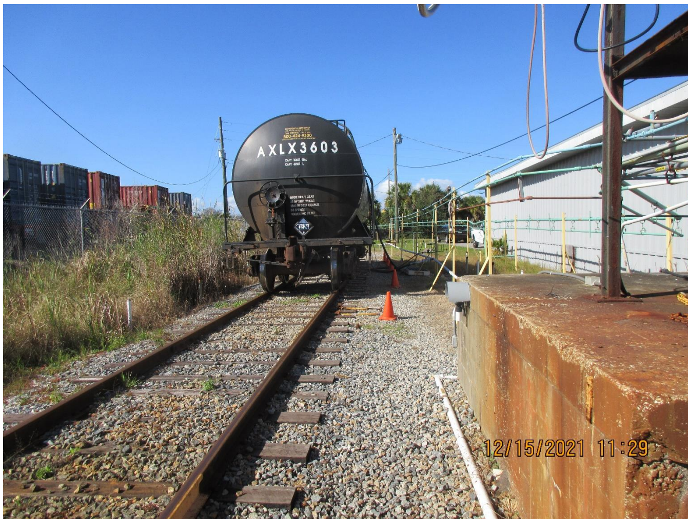
Photo 18 – Railcar Off-Loading Area
