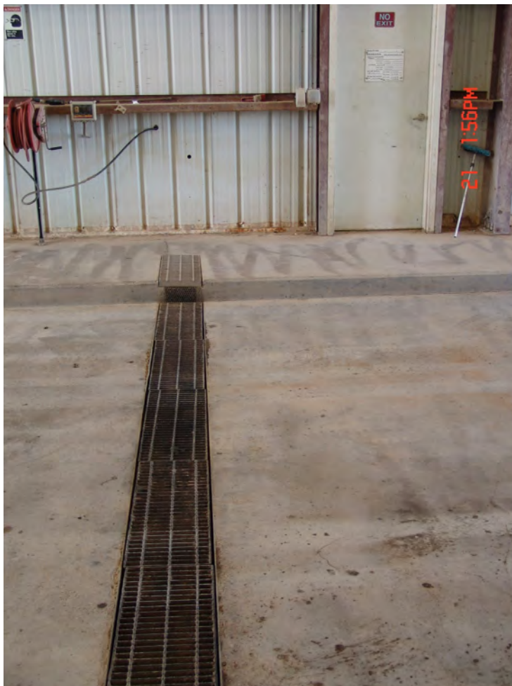
Wash rack at Material Test Directorate bldg. 2780 drainage trough.
