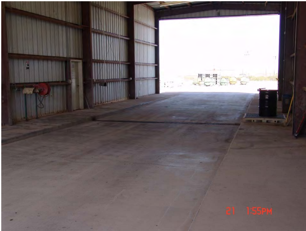
Wash rack at Material Test Directorate bldg. 2780 looking east.
