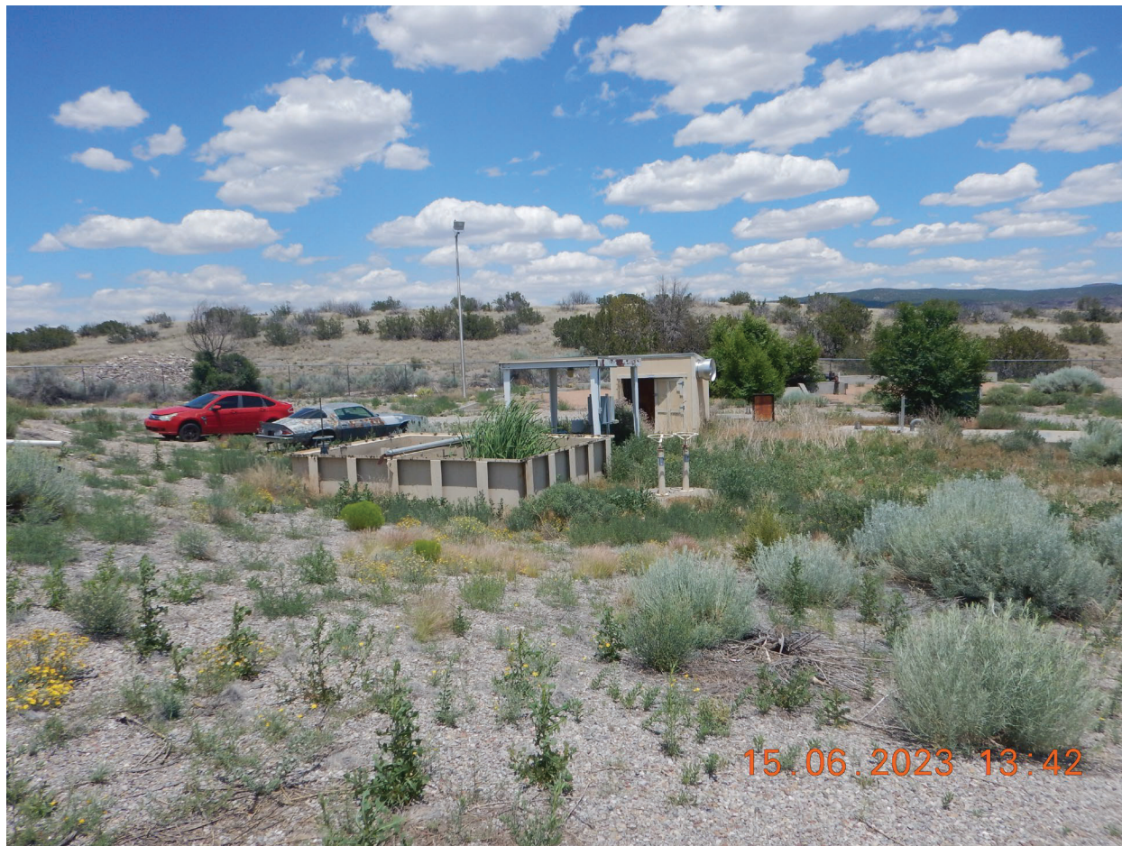
View of additional decommissioned process treatment equipment situated along the eastside of the facility. (DSCN 2604). Photographed by D. Esparza.
