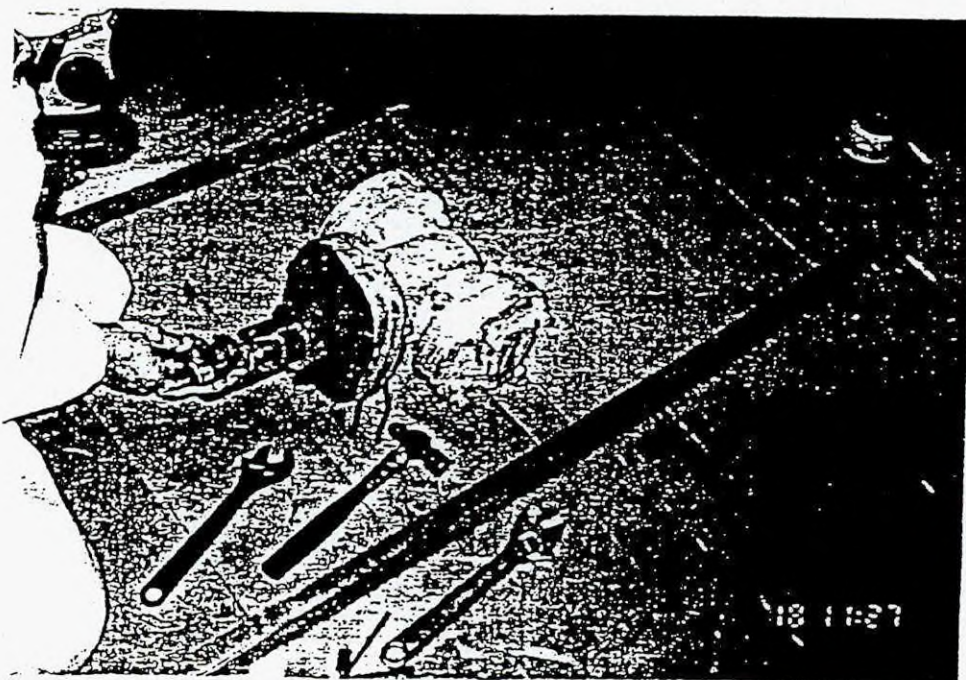
Figure 4. Removing packing.
