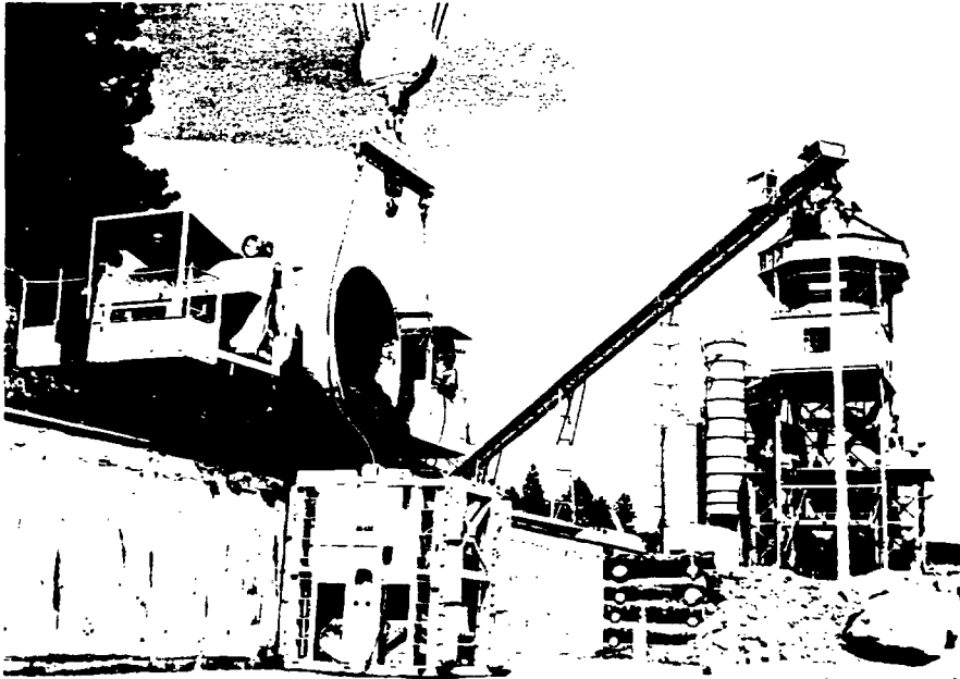
Concrete bucket dock at the Box Canyon Dam project. The electric "goose car" is dumping three inch mass concrete into an 8 cubic yard bucket which travels by cableway to one of the main blocks in the dam. In the background is the concrete mixing plant.
