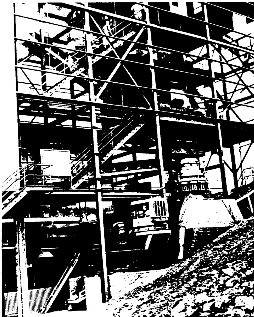
A closeup of the magnetic separating plant at Buena Vista mine in Nevada. At the top level of the plant is the primary magnetic separating equipment. Below are the secondary and tertiary crushers. The plant was constructed and operated by Minerals Materials Co. prior to its being sold to U.S. Steel in 1958.
