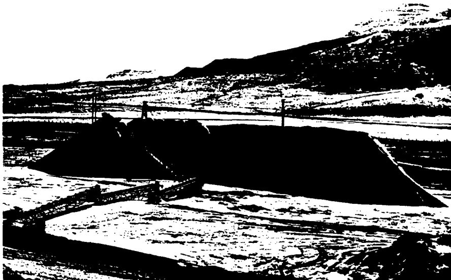
Conveyor system stockpiling products from the crushers at California Portland Cement Co.'s quarry. The finished material is loaded on trucks and hauled to their cement plant 14 miles away.
