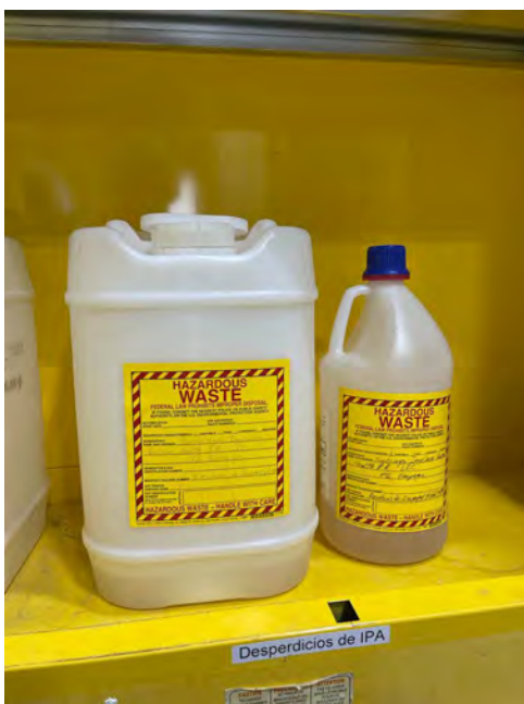
Photograph 5: Facility's corrective action – F6 SAA with a 5-gallon container of isopropyl alcohol marked and/or labeled with the words “hazardous waste” and with an indication of the hazards of the contents.
