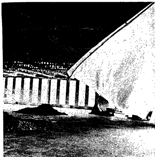
Figure 5. Floor of building after spray application. Note piles of waste asbestos-containing materials and flapping tarpaulins, inadequately secured.
