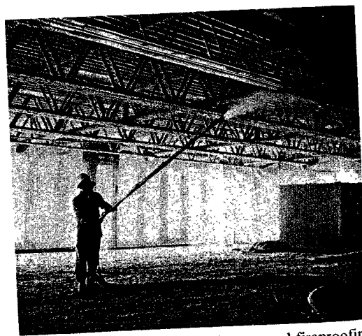
Figure 2. Applicator applying sprayed fireproofing containing asbestos. Note waste material on floor. Worker is wearing respiratory protection, inadequate for such intense exposure.
