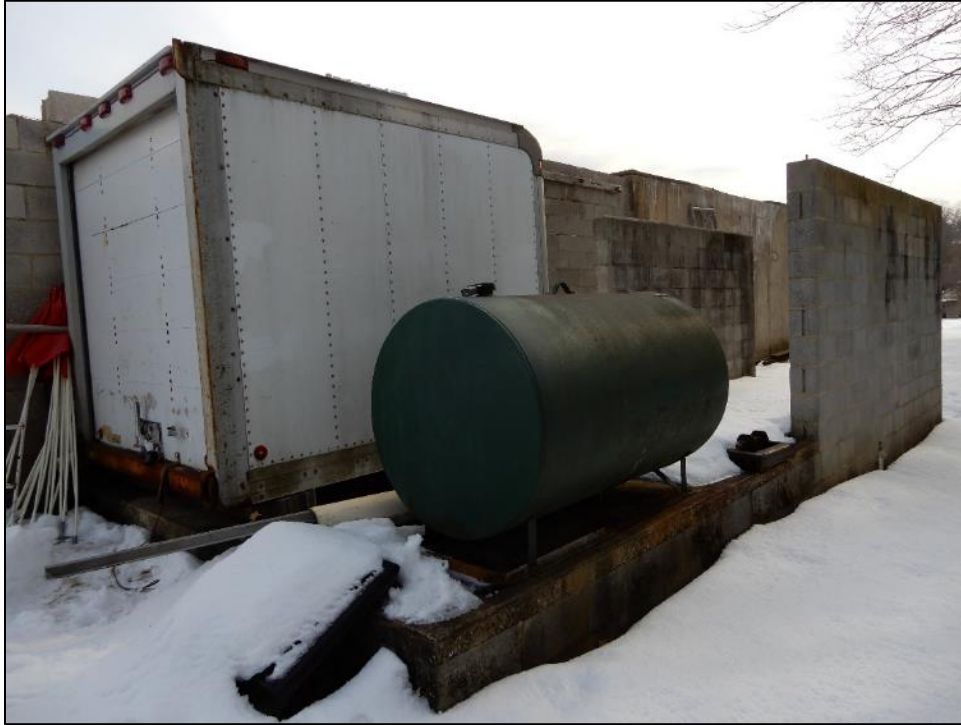
Photograph 5. View, facing southeast, of the used oil storage tank located on the western side of the property. The tank had a volume of approximately 150 gallons; it was not double-walled or located within secondary containment.
