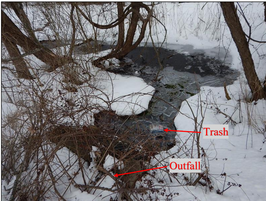
Photograph 29. View of partially frozen water pooled in front of the outlet from the stormwater basin into the wetland area located east of the BMP. Note trash observed near the outlet.
