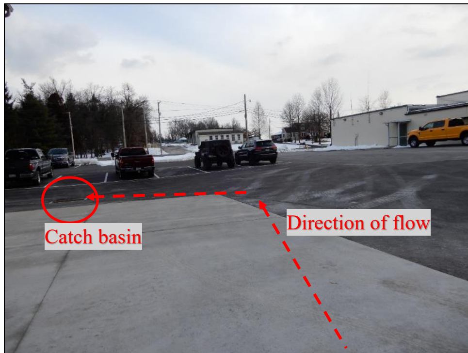
Photograph 2. View, facing east, of the new parking lot area north of the existing Maintenance Building.
