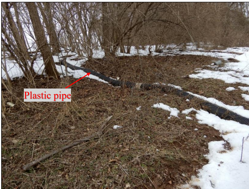
Photograph 34. View, facing northwest, of the plastic pipe from the apartment complex parking lot leading to the stormwater basin.
