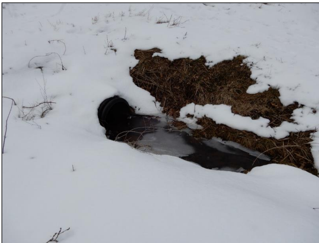
Photograph 33. Additional view of the outfall to Hartman Run.
