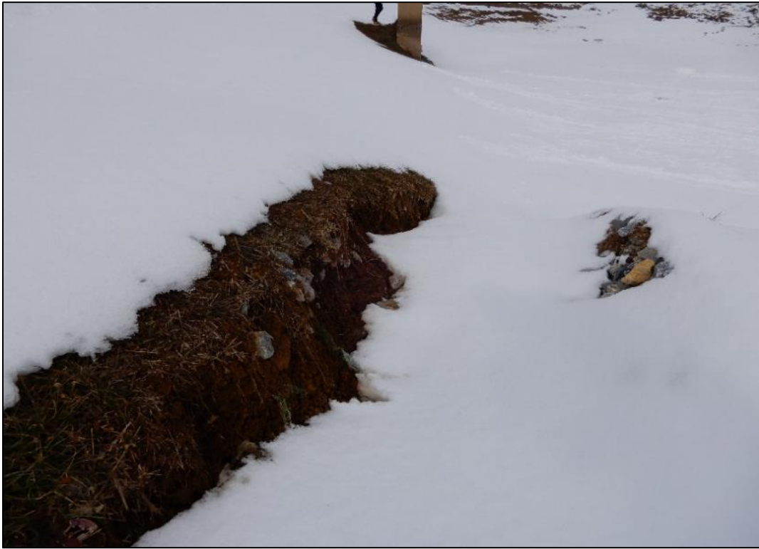
Photograph 42. Alternate view, facing northeast, of the erosion observed in the center of the stormwater basin.
