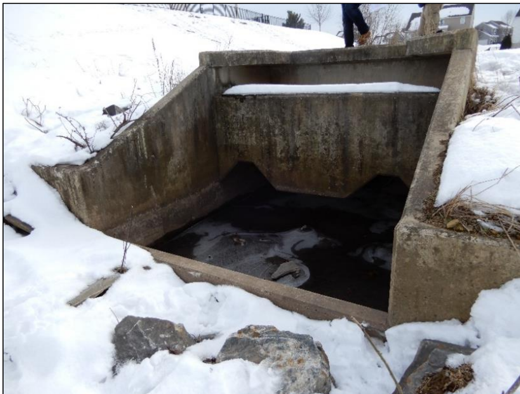
Photograph 37. View, facing south, of the dual inlet structure at the southern end of the basin.
