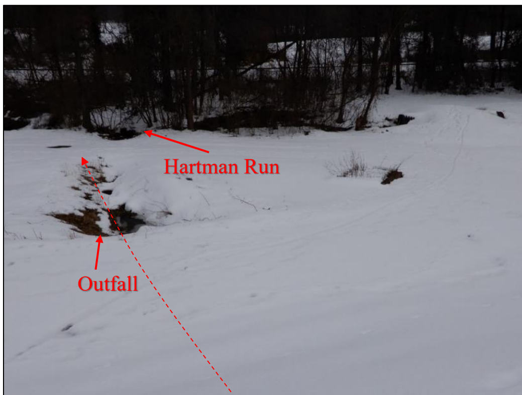
Photograph 32. View, facing east, of the outfall structure and Hartman Run.
