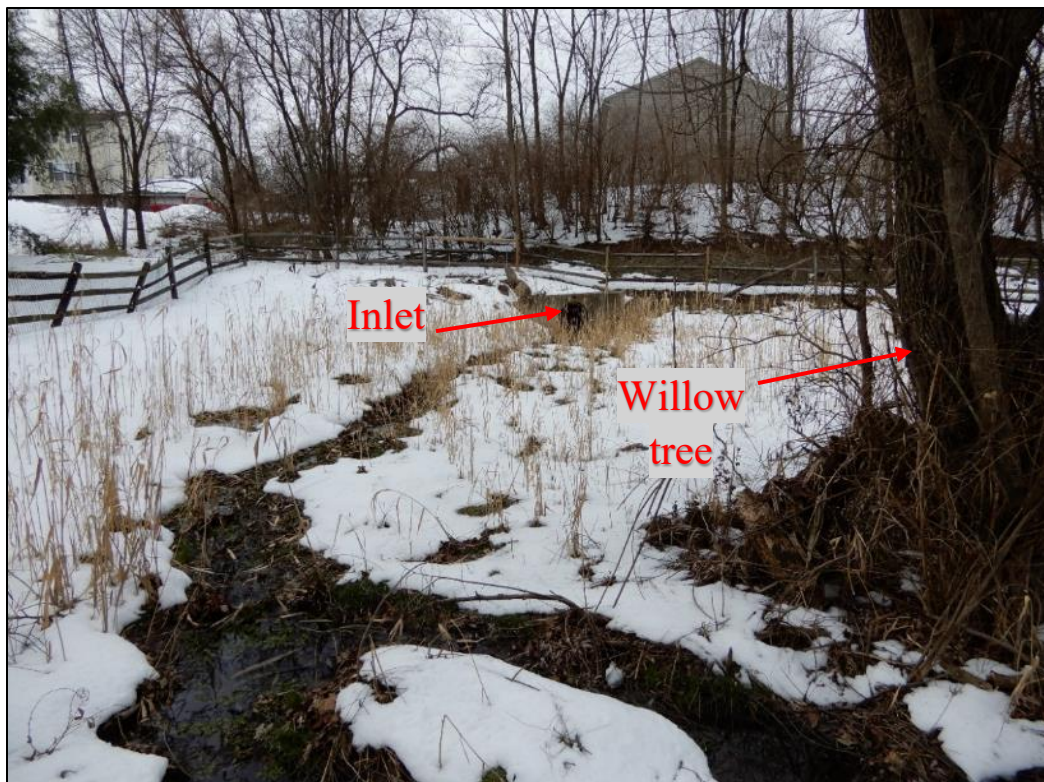
Photograph 31. View, facing southeast, of the inlet in the southeastern end of the stormwater basin. Also note the vegetation and willow tree.
