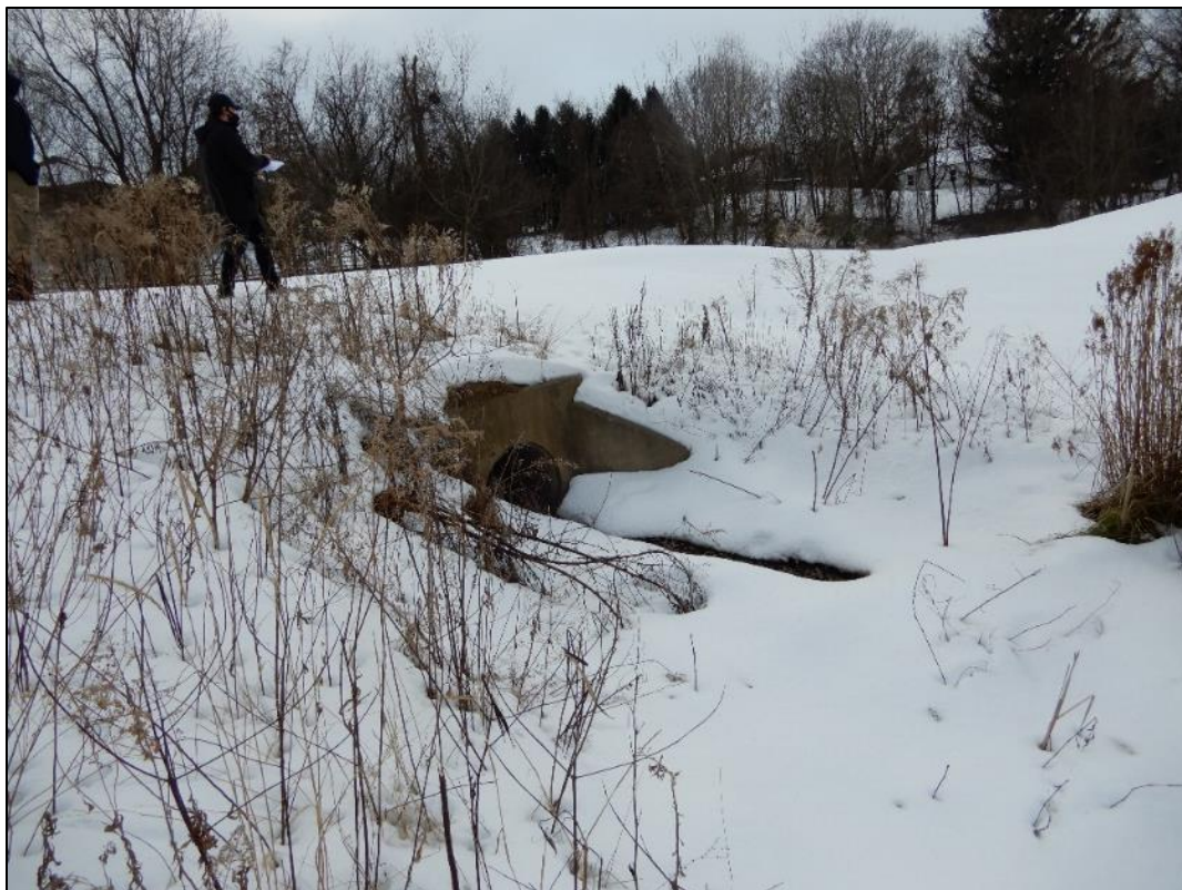
Photograph 45. View, facing east, of the inlet into the stormwater basin.
