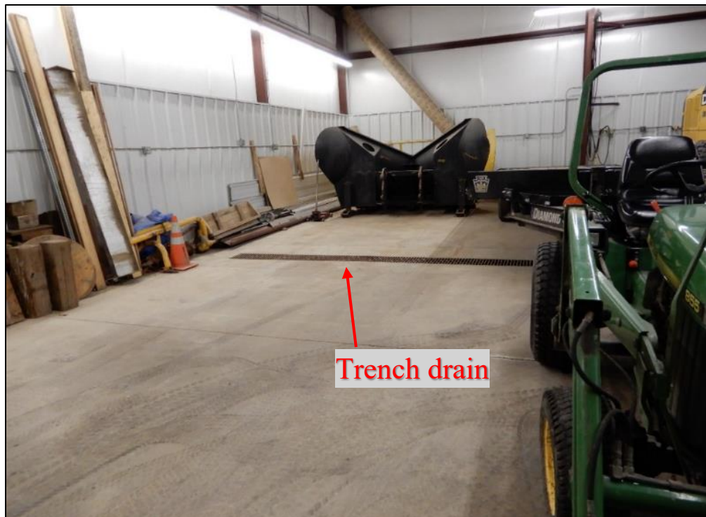
Photograph 13. Additional view of the trench drain that stretches the length of the garage.
