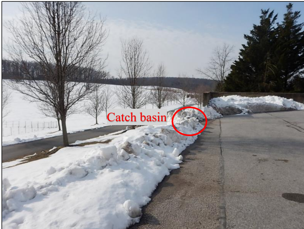
Photograph 9. View, facing southwest, of a catch basin covered in snow on the southern border of the property. The runoff from the impervious pavement in front of the garage on the southern portion of the property drains to the basin, then to an infiltration bed on the south side of the parking lot.
