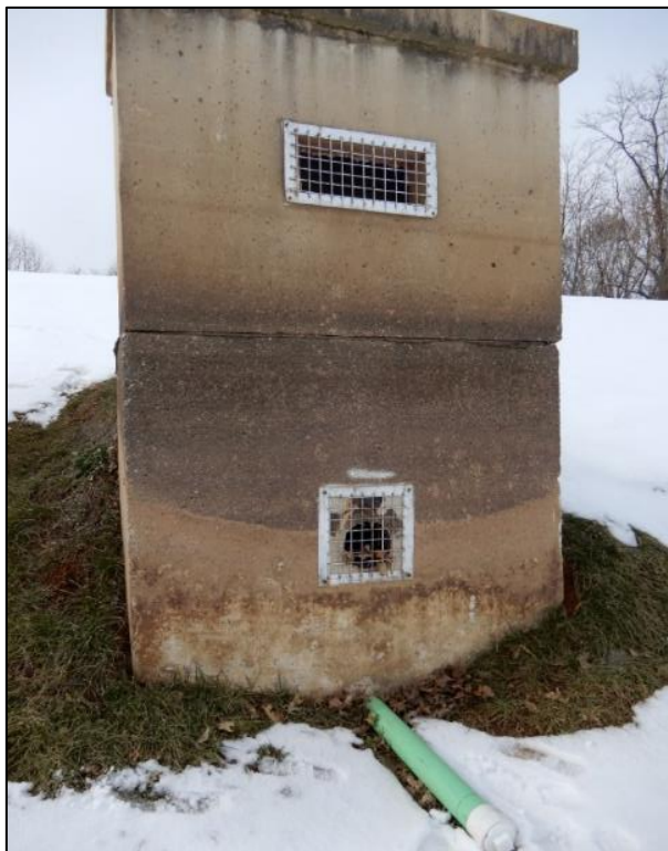
Photograph 39. View, facing west, of the concrete riser outlet structure.
