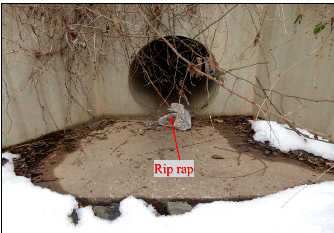
Photograph 47. View of the outfall to the tributary to Musser Run. Note rip rap was observed at the outfall.
