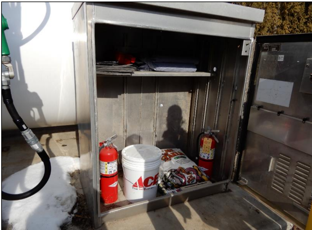
Photograph 17. View of the spill kit stored at the fueling station.
