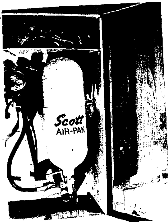
Fig. 9-6. Wall-mounted storage cabinet for a SCBA.
