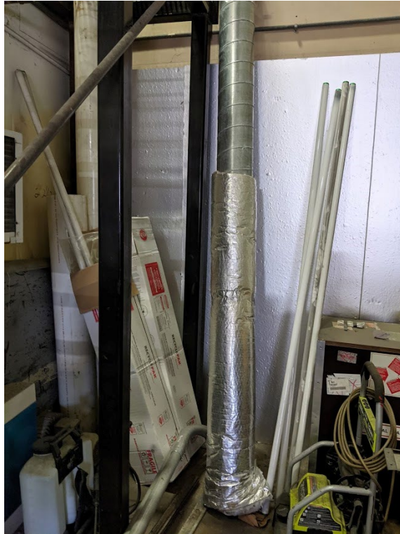
Photograph 17 of 21: Maintenance Parts Room – Universal Waste Storage Area
