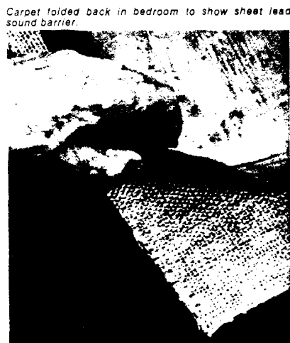
Carpet folded back in bedroom to show sheet lead sound barrier.
