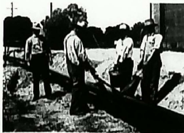
APPLICATION OF "McEVERLAST" ELECTROLYSIS PROOF COATING TO SINK GAS MAIN OF SOUTHERN CALI- FORNIA GAS COMPANY
