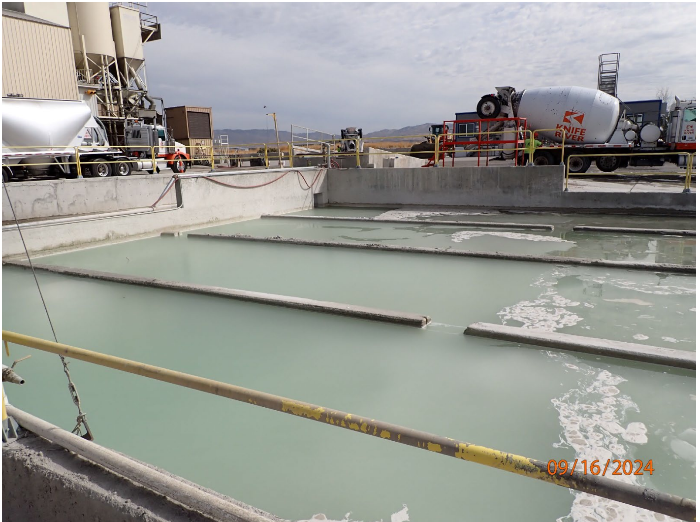
Photo 1 - Concrete washout area
