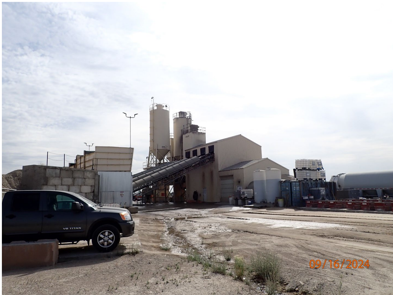
Photo 3 - Ready-mix cement plant
