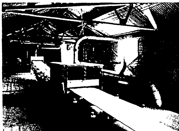
Dust-filter installation used to exhaust a belt conveyor in a modernized cement plant in Canada. Observe the piping system through which the dust is drawn off
