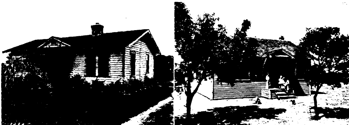
At left, a home at Lemon City, Fla., and at right, a new Texas farm house, both built under the Extension Service supervision to rehabilitate poorly-housed families. White lead plays a major part in rural re-housing such as this
