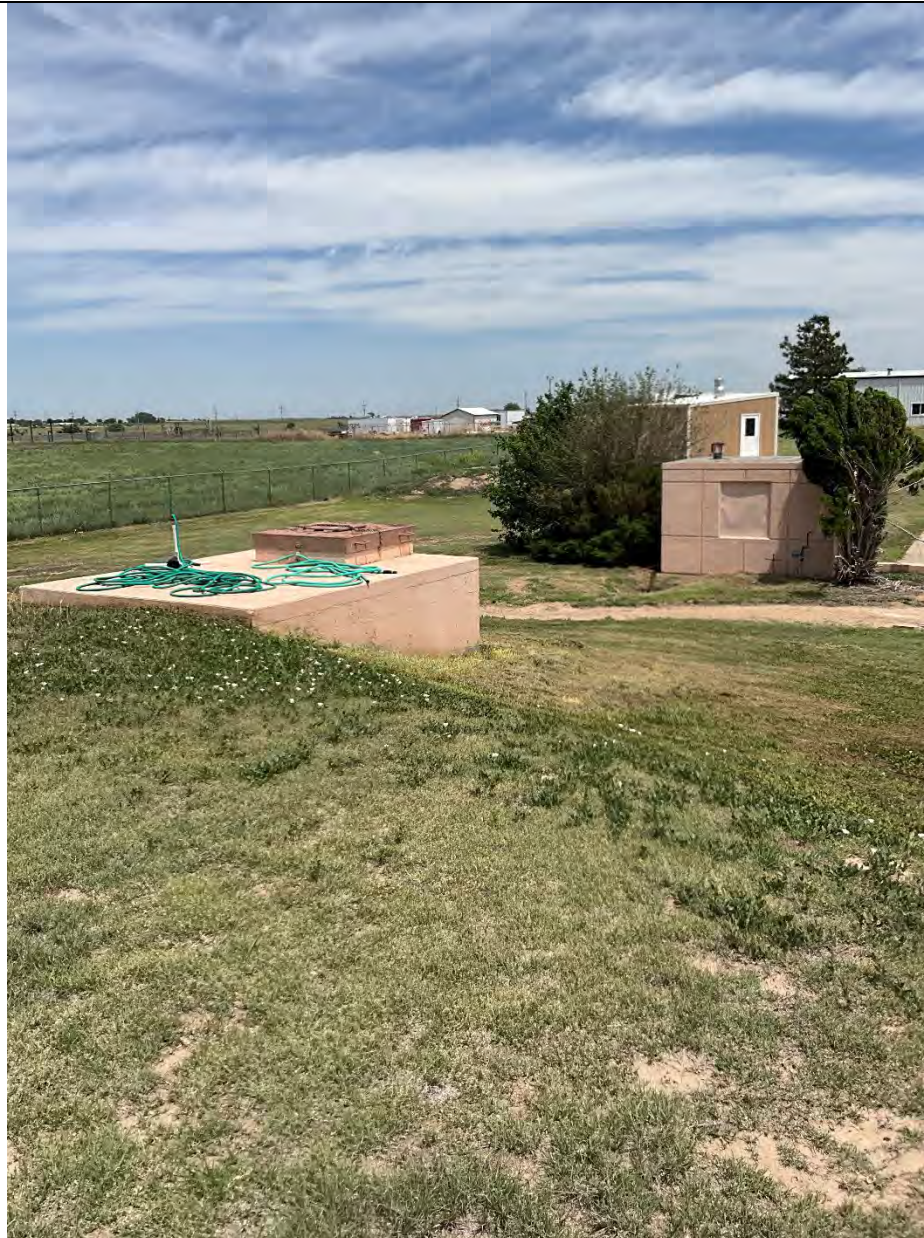
Station #4 – View of the sand collection pit access hatch prior to the GST.
