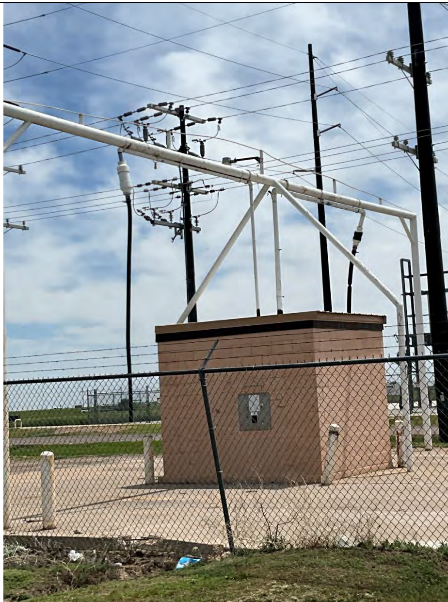
Bulk water filling point at Station #4. Note the air gap is twice the diameter of the fill pipe
