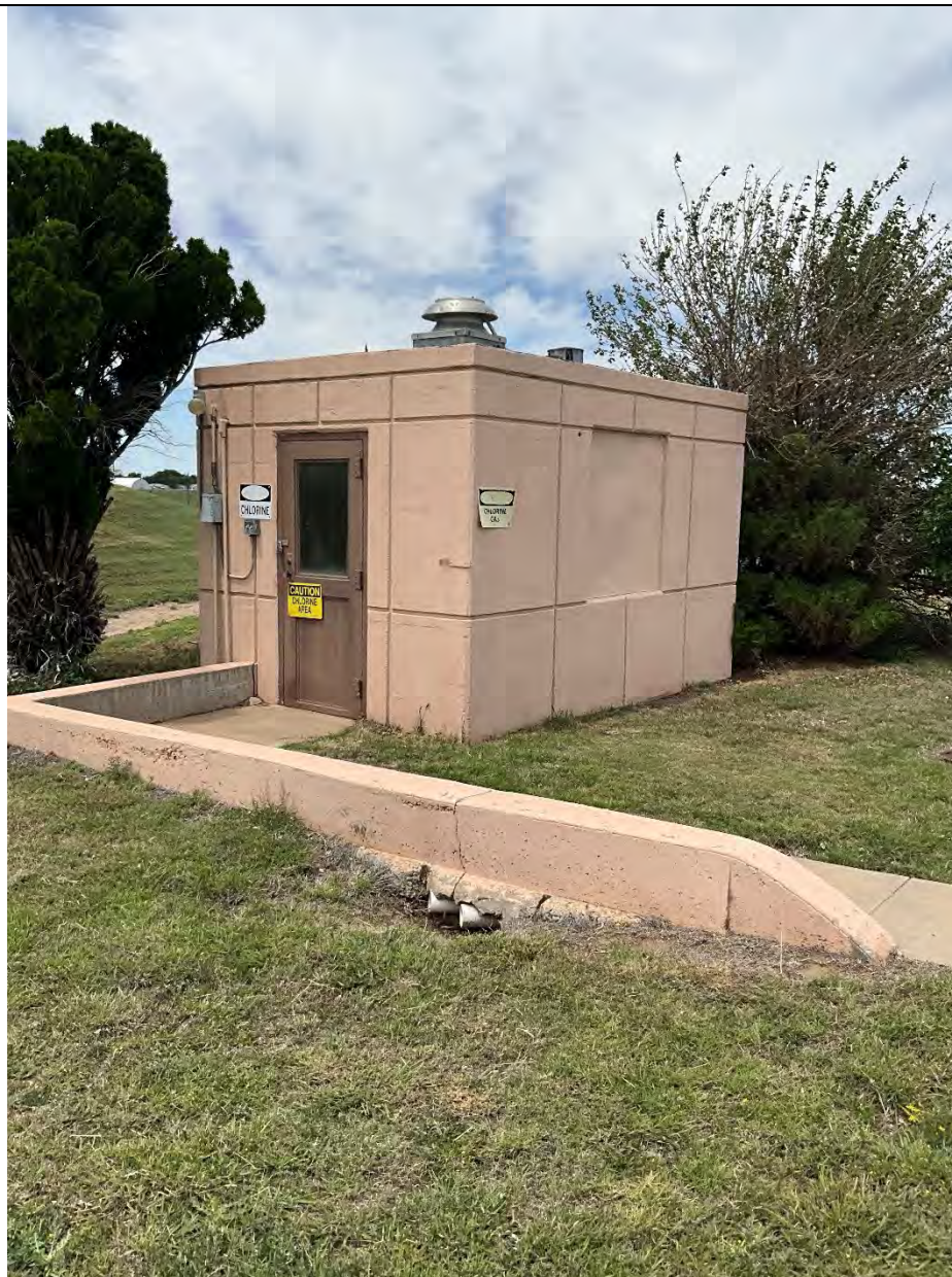
Station #4 – Chlorine gas storage building with secure door, sound structure, and chlorine exhaust on the roof of the structure.
