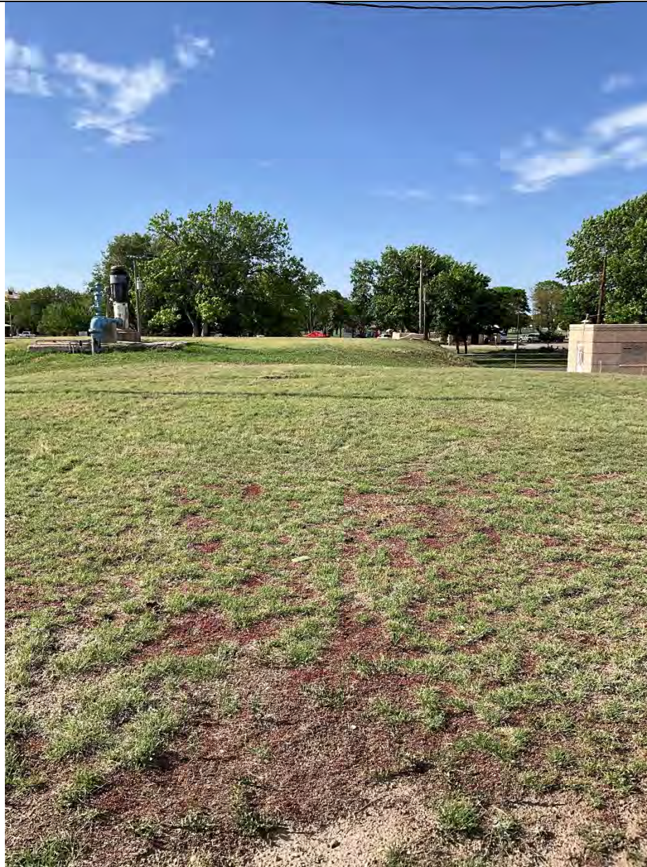
Station #1 – View of the top of two GSTs and the high service pump and chlorine storage building in the background; note no vent on either of the GSTs
