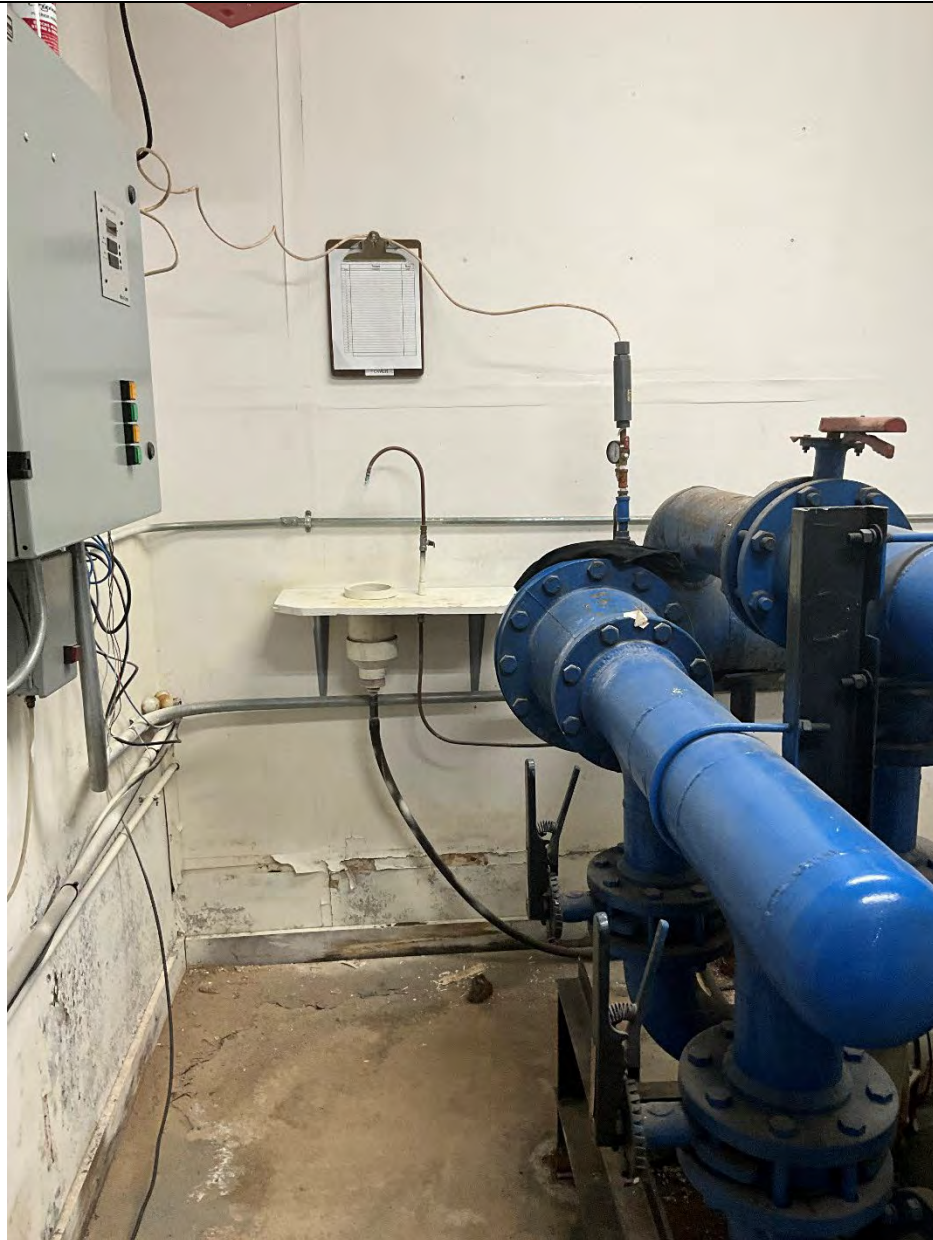
Water tower sampling location and inspection log
