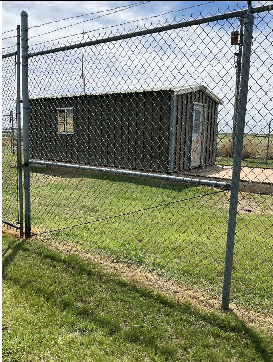
Well #3-3 view of exterior of building and security fencing
