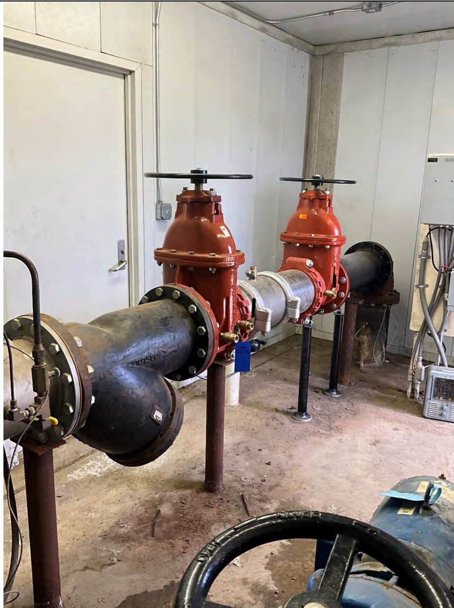
Consecutive connection with National Beef – backflow prevention device protecting the connection.
