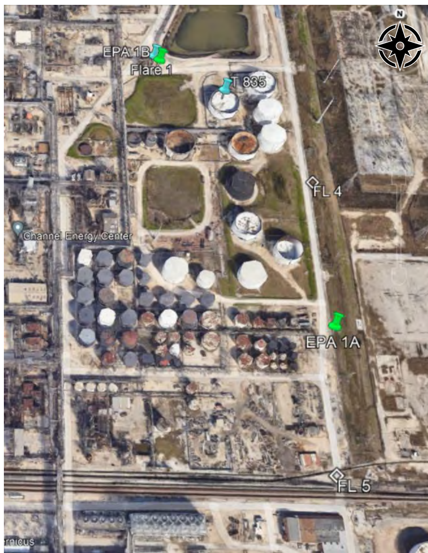
Figure 2. EPA 1 eGC Site Overview
