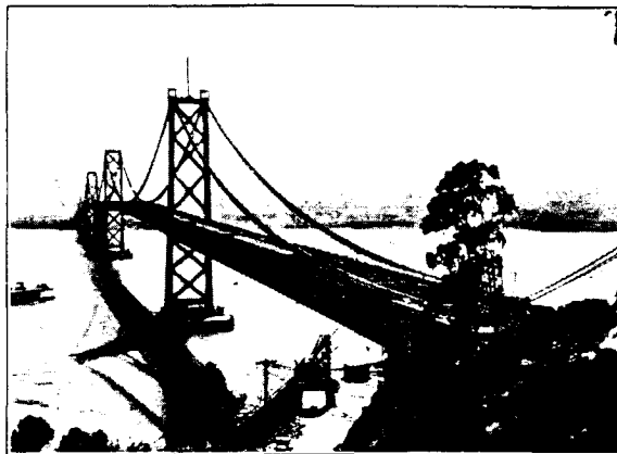
Suspension spans of the San Francisco-Oakland Bay Bridge on which lead wool is used to calk suspender rope saddles and red lead protects the steel.
