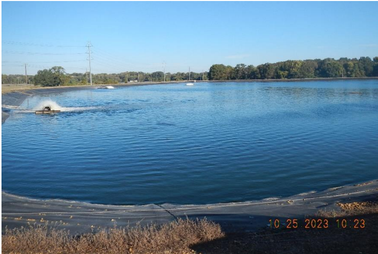
Photo 1. Cell 2, operational aerators.
