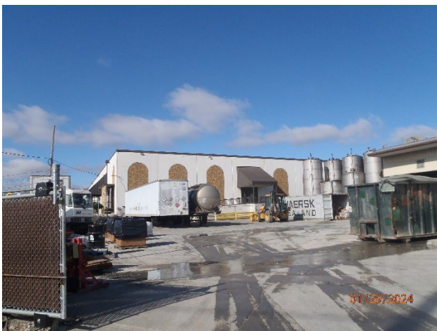
Picture 3 – Inbound Staging Area
