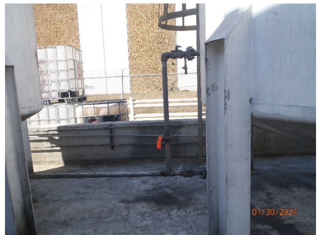
Picture 24 – Tank System 1 Tank B7 flange leak repaired
