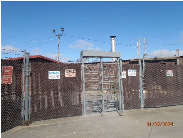
Picture 1 – Perimeter fence and signs
