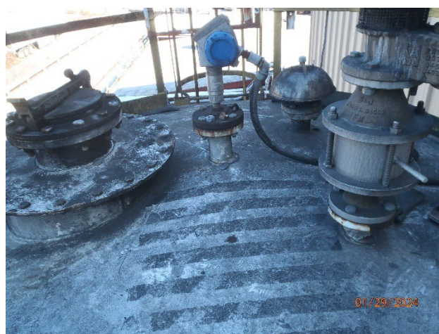
Picture 51 – Tank System 2 top of tank
