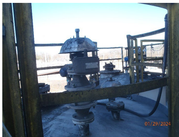
Picture 50 – Tank System 2 top of tank
