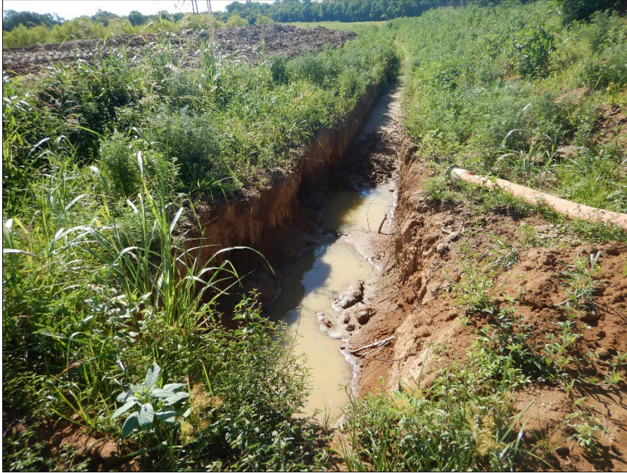
Photograph 11. View, facing southeast, of a manmade trench used for the discharge of the water pumped from the sediment basin.
