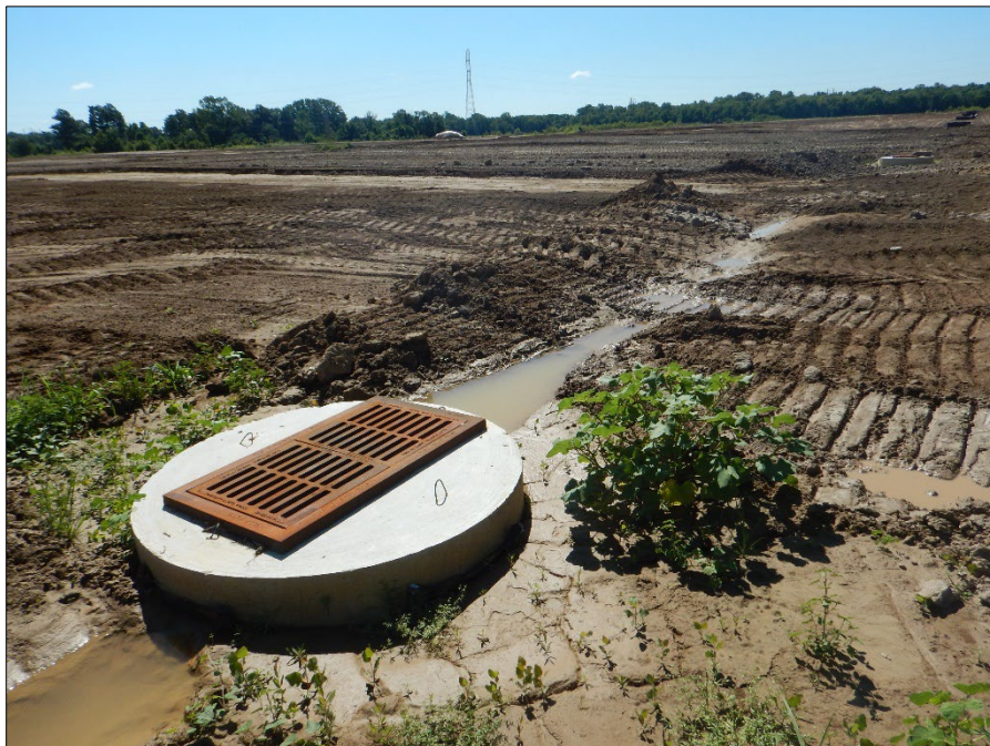
Photograph 14. View, facing east, of a raised inlet in the center of the Site.
