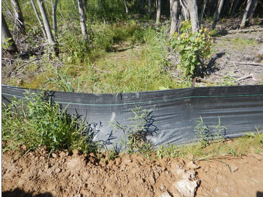
Photograph 13. View, facing southwest, of sediment and vegetation against the perimeter silt fence in the southern portion of the Site.
