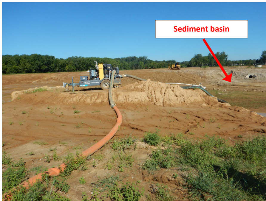
Photograph 10. View, facing southwest, of a pump removing water from the sediment basin.
