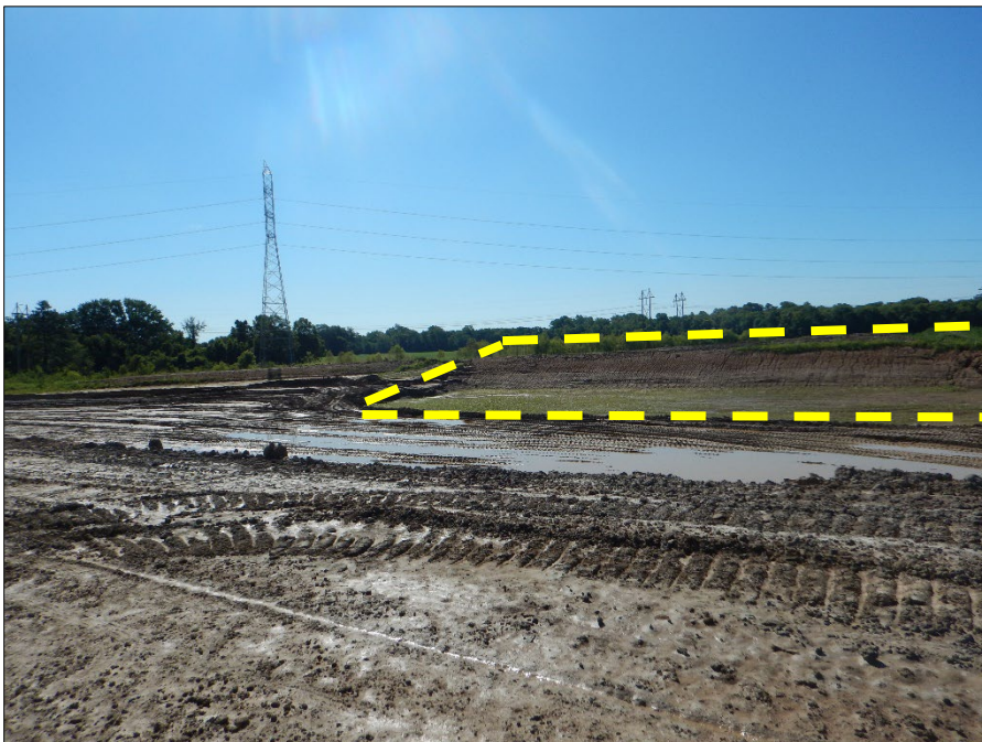
Photograph 4. View, facing southeast, of a disturbed area and sediment basin (dotted yellow lines) in the southeastern portion of the Site.
