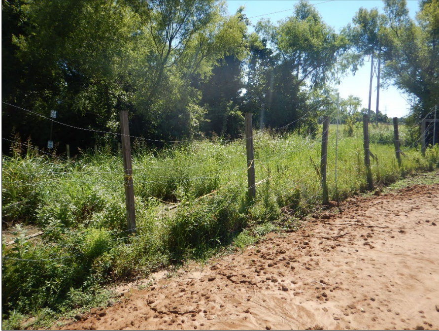
Photograph 25. View, facing northeast, of the northern boundary of the Site. According to the Site EPSC Plan, the Site should have silt fence along the northeastern boundary of the site. However, at the time of the inspection, no silt fence was present.
