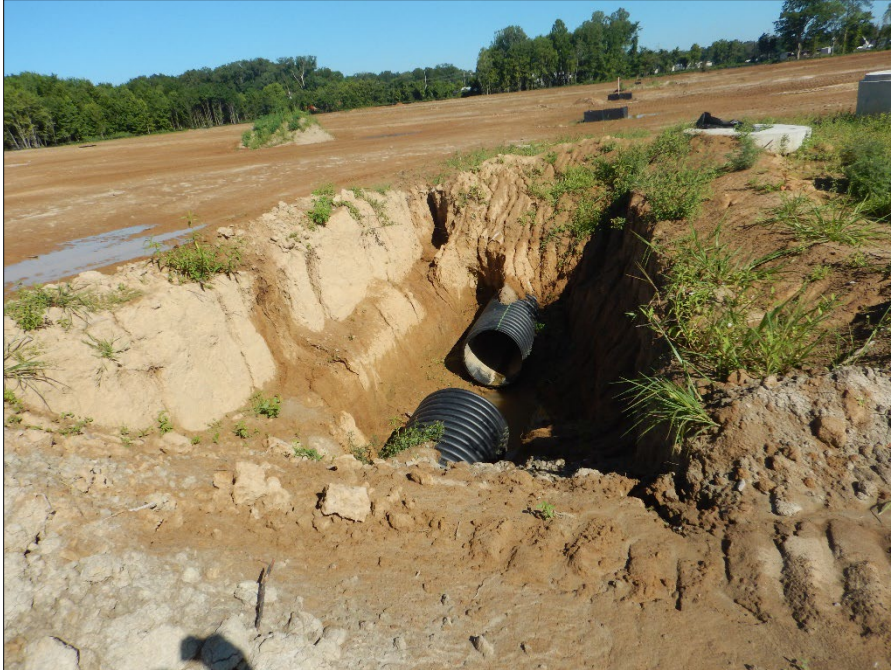
Photograph 3. View, facing northwest, of corrugated piping that was being installed in the southern portion of the Site.
