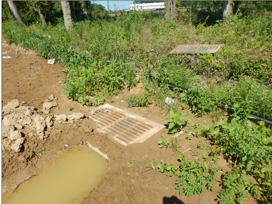
Photograph 23. View, facing southeast, of an inlet without any inlet protection to prevent sediment intrusion.
