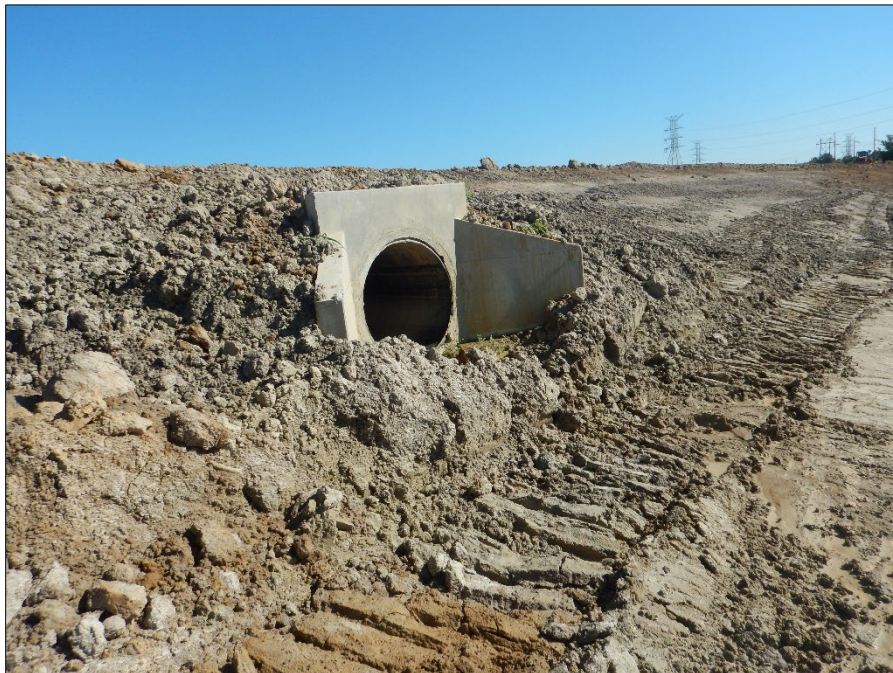
Photograph 6. View, facing north, of a headwall and pipe leading into the basin shown in Photograph 5 . At the time of the inspection, the stormwater piping had not been connected to this basin but had been connected to others.
