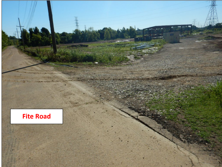
Photograph 1. View, facing northeast, of a Site entrance/exit off Fite Road. The entrance/exit did not have sediment controls, and sediment track out was observed leading from the Site onto Fite Road.
