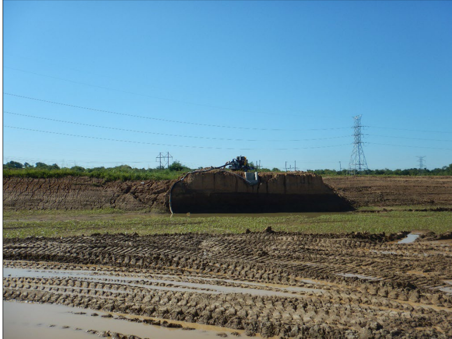
Photograph 7. View, facing southeast, inside the sediment basin shown in Photograph 5 .
