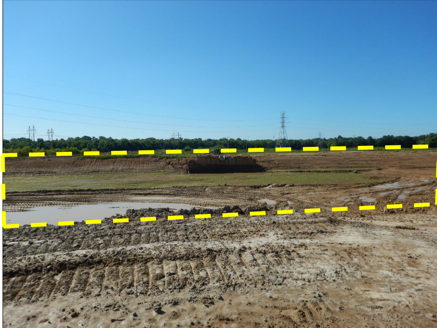
Photograph 5. View, facing southeast of the sediment basin in the southeastern portion of the Site. At the time of the inspection, the basin had not been stabilized, but was being utilized by the Permittee as a temporary basin during construction.
