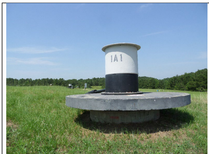
Landfill Section 1. The inspector observed pump enclosure 1A1. Photograph 15 taken at 11:24 a.m.
