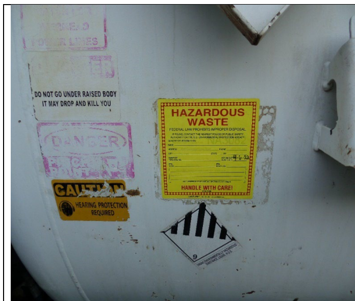
Central Tank Farm. The inspector observed the 3,300-gallon vacuum truck not marked with a toxic hazard indicator. Photograph 5 taken at 10:27 a.m.
