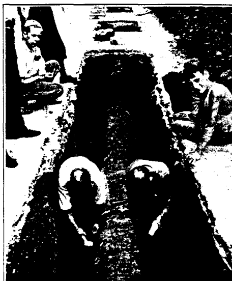
DENNIS PHOTO SERVICE CO. Bethlehem, Pa., water department team calking lead joints in new cast iron bell and spigot water main.
