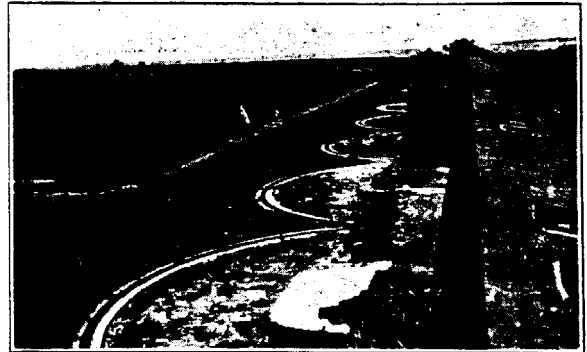
Fort Pulaski, Georgia, showing earth covered lead roof.
