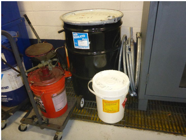
Photo 11: The third SAA at the Building 4430 Vehicle Maintenance Area. One 5-gallon container for accumulating hazardous waste used aerosol cans as hazardous waste.
