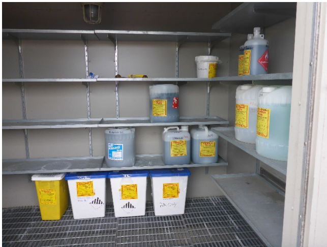
Photo 8: Approximately sixteen containers of hazardous waste, each with a capacity of 5-gallons or less, on shelving within a HazMat storage building / Flammable storage shed at the CAA.
