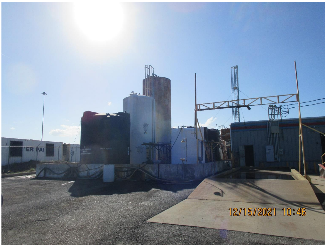
Photo 5 – Tank farm and bleach manufacturing area
