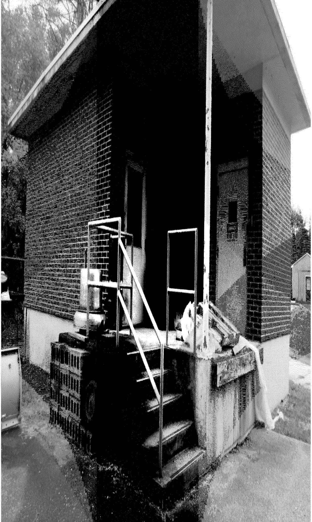
Warner Village WWTF 55 W Joppa Rd. Warner, NH CWA NPDES Inspection October 18, 2023
