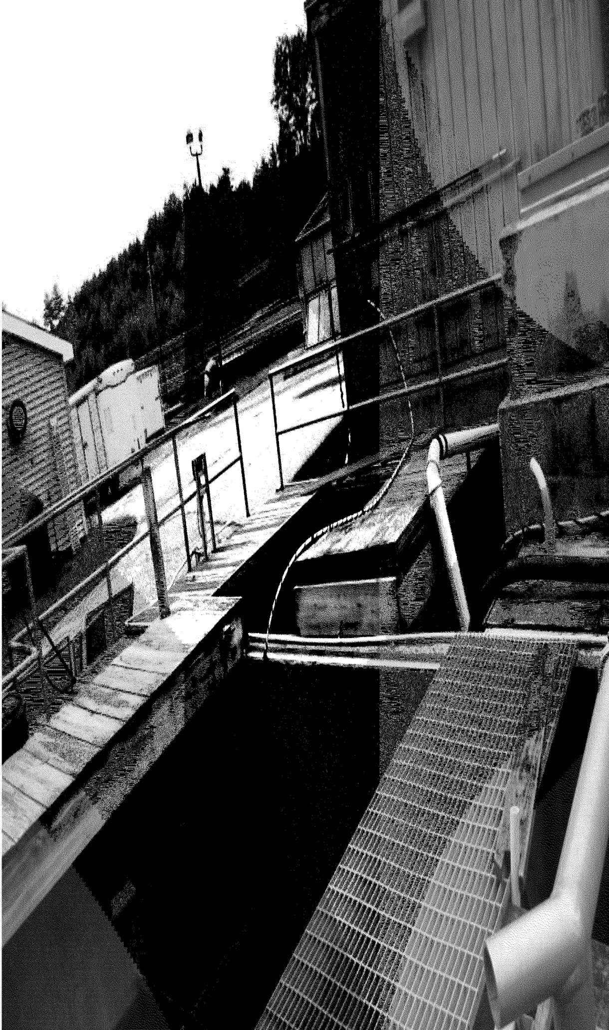
Warner Village WWTF 55 W Joppa Rd. Warner, NH CWA NPDES Inspection October 18, 2023
