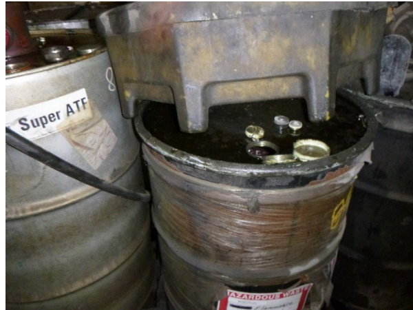
Photo 24: Vehicle Maintenance Building SAA.
