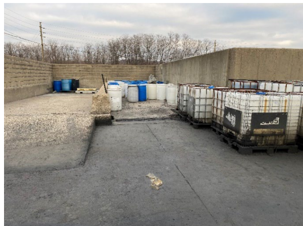
Photo 41: Used Oil Pad.
