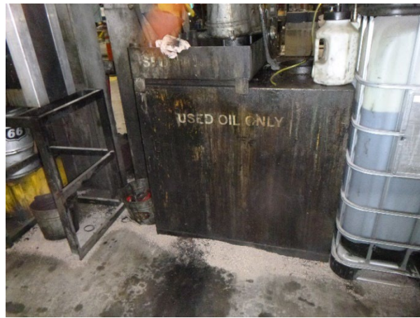
Photo 23: Used Oil Tank.
