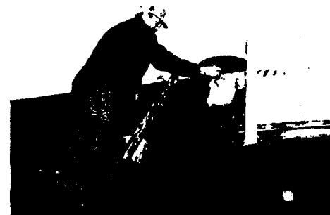
PLANT PAINTER, W. Wagner applies protective finish to about 400 feet of new shelter for the belt conveyor at the Bound Brook Plant.
