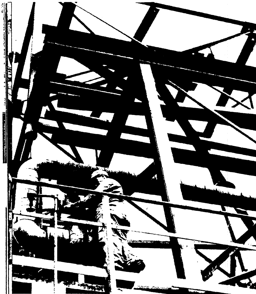
ED. COLEMAN, CHICAGO, STANDS ON A NARROW CATWALK HIGH ABOVE THE GROUND TO CHECK A VALVE AT THE PHTHALIC ANHYDRIDE PLANT.
