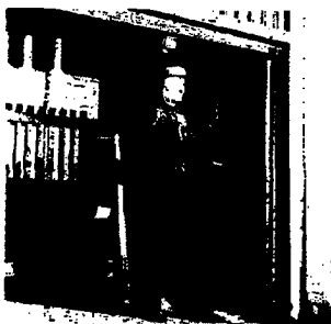
ELEVATOR OPERATOR, J. Segos, is a busy man at the Sherwin-Williams Cleveland Plant.
