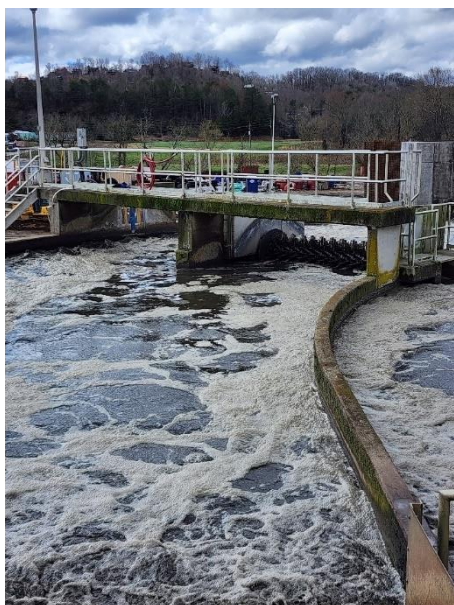
Photo 3: Oxidation ditch paddles missing/out of service. Photo 4: Floating aerators in oxidation ditch.
