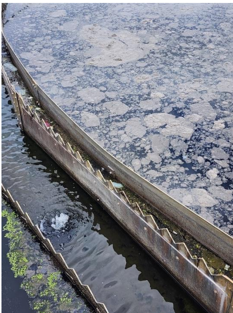
Photo 7: Floating grease and duckweed on clarifier #1.
