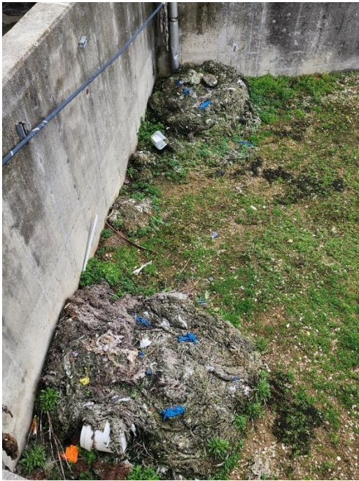
Photo 5: Solids on ground between clarifiers.
