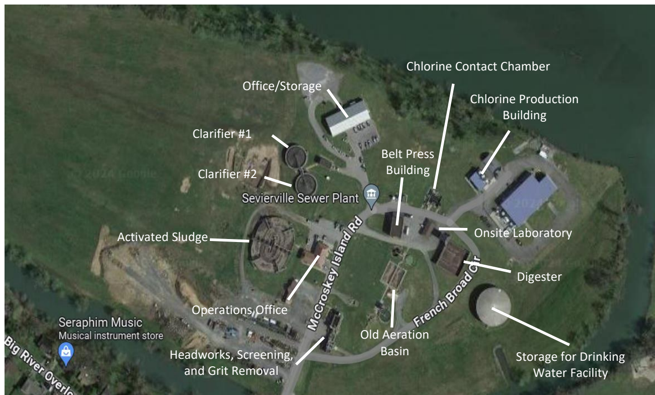
Figure 1: Aerial View of the Sevierville Sewage Treatment Plant
