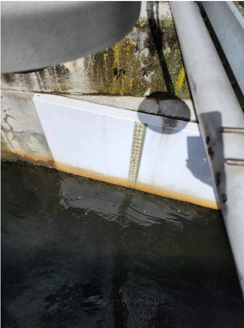
Photo 13: 3-foot parshall flume staff gauge.
