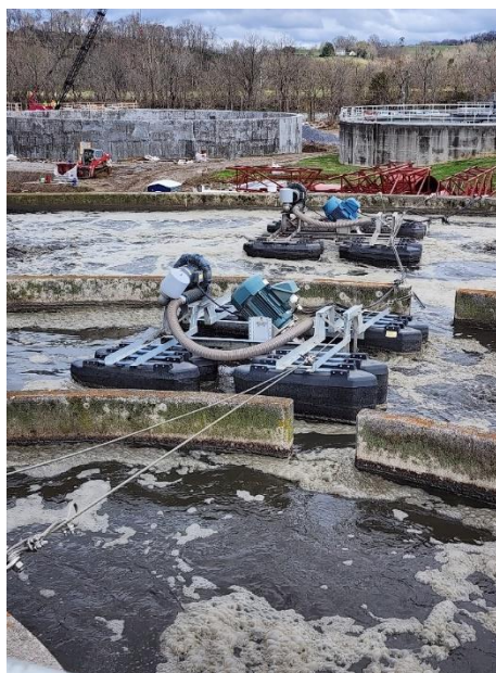
Photo 3: Oxidation ditch paddles missing/out of service. Photo 4: Floating aerators in oxidation ditch.
