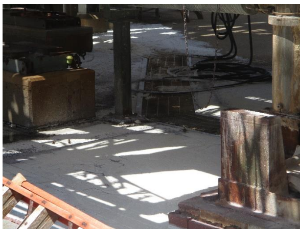
Picture 1: PTA Unit #5
