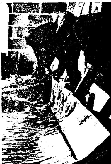
2. Crimping pigeared corner. Hole for drain already cut out.
