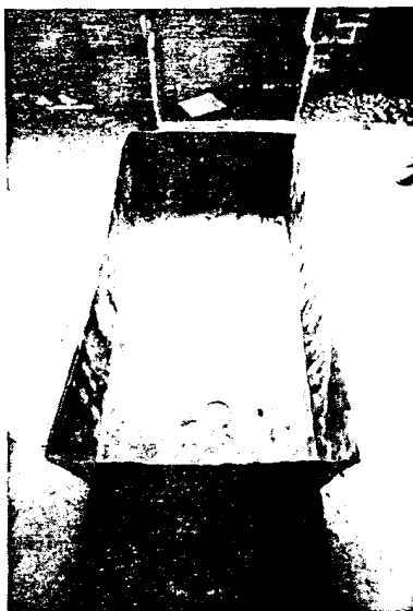
5. Completed pan before installation in shower room.
