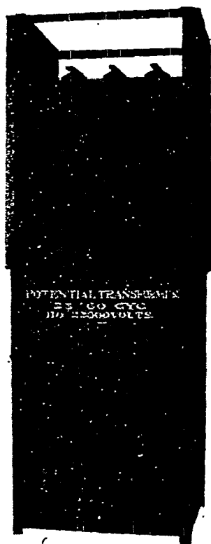
22,000 volt potential transformer cage, Schenectady Works.
