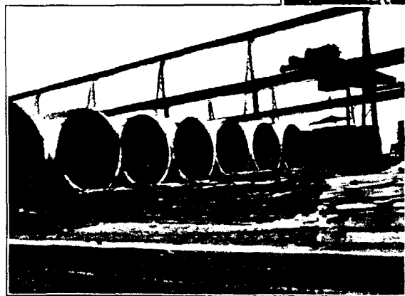
Installing huge concrete pipe for Metropolitan Water District of Southern California project and, below, concrete pipe in the manufacturer's yards with piles of special lead gaskets for jointing it.
