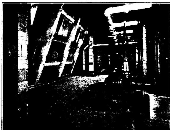
Tank room in the Court House tower. The floor is completely covered with sheet lead with "burned" seams. The lead turns about 6 in. up walls and columns.
