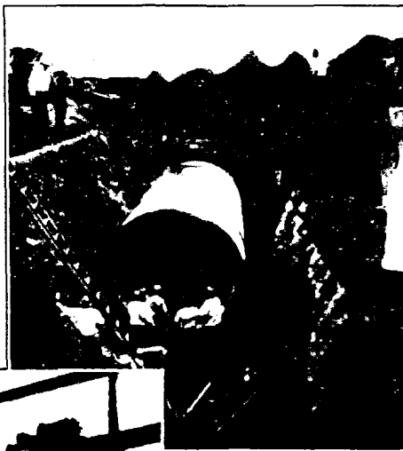
Installing huge concrete pipe for Metropolitan Water District of Southern California project and, below, concrete pipe in the manufacturer's yards with piles of special lead gaskets for jointing it.
