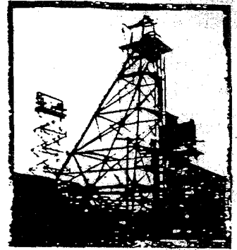
Head frame at mine shaft
