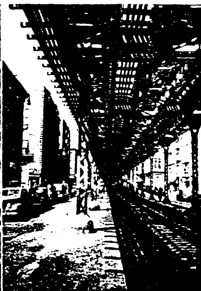
View along 3rd Ave., several shades lighter as a result of the repainting.
