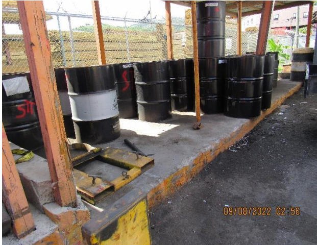
IMG 503 -Lubricant and chemical storage area. No containment to capture spills and leaks onto concrete base. Will be washed-off by stormwater runoff flow.
