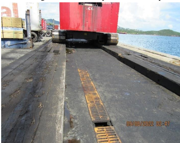
IMG 495- Evidence of oil and grease residue open to all environmental conditions. Dock graded to allow stormwater to drain towards inner yard and the catch of spills and leaks of oil and grease in yard area basins. IMG 492- Container transport vehicle in operation in dock area and inner yard. Increased possibilities
