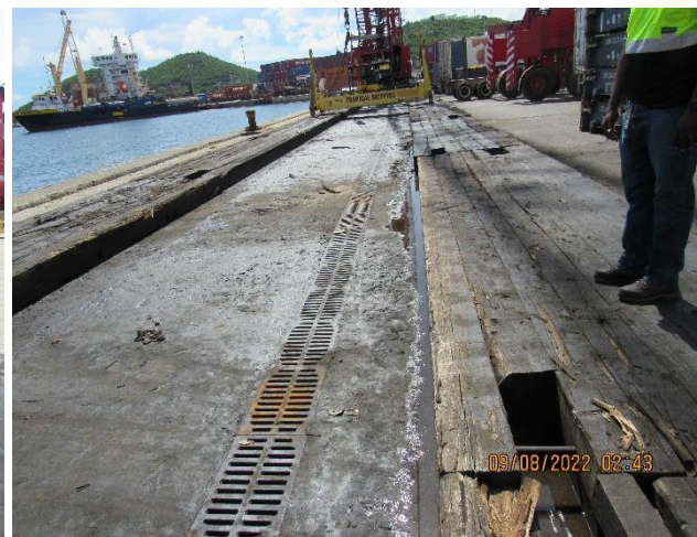
IMG 489- Crain staged on dock platform for loading and unloading cargo. Drain collects stormwater runoff, oil and grease leaks and spills installed in place. IMG 490- View of the drain along the entire dock bulkhead.
