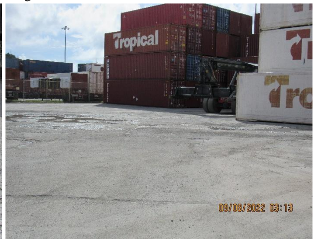
IMG 519 -View of Tropical's MT Yard area that drains into the single stormwater catch basin.
