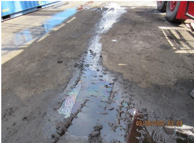
IMG 513 -Evidence of oil and grease residues draining into inlet of a submerged Oil/Water Separator in operation at the Facility.
