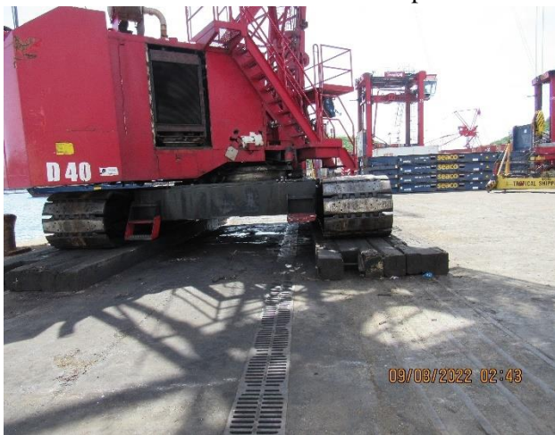
IMG 489- Crain staged on dock platform for loading and unloading cargo. Drain collects stormwater runoff, oil and grease leaks and spills installed in place. IMG 490- View of the drain along the entire dock bulkhead.
