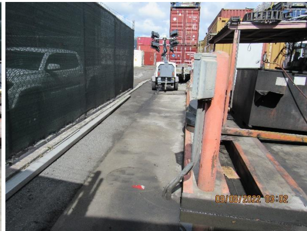
IMG 512 -Evidence that used oil residue washed-off by stormwater runoff flow towards stormwater catch basins in the central area of the Facility.
