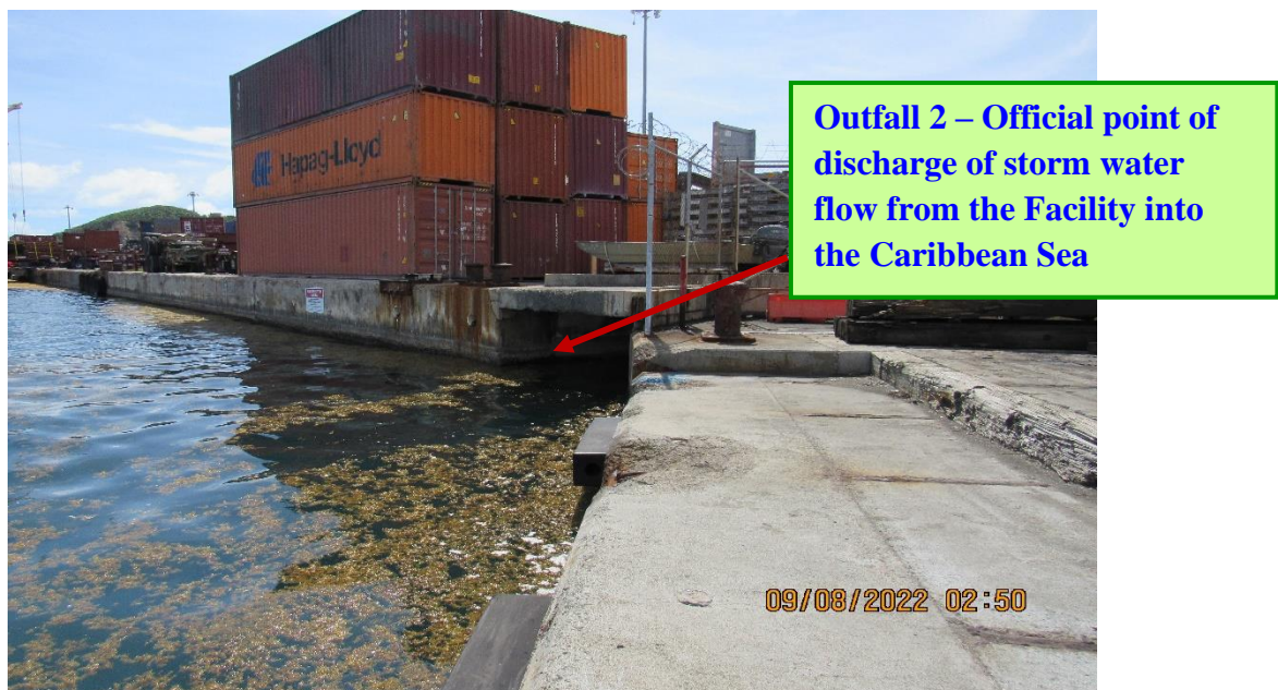
IMG 496 -Discharge point of a stormwater channel that traverses the Facility. Stormwater runoff from Tropical's MT Yard drains into the channel before final discharge into the Charlotte Amalie Harbor.
