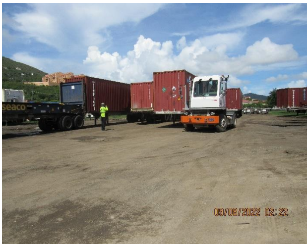
IMG 475 -Front area of the Cancryn Field section occupied by Tropical. On-going activity observed, with no erosion control and soil retention installed.
