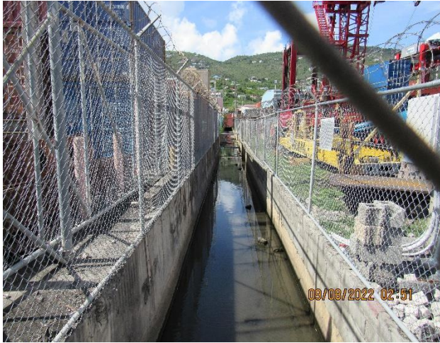
IMG 498 -Large stormwater drainage canal that runs through Tropical, north to south, and drains into the Bay.
