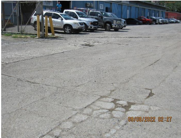
IMG 479 -A stormwater catch basin of stormwater drainage system in the Crown Bay port area.
