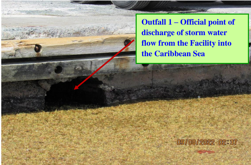
IMG 486 -Discharge point where storm water from the Field and Warehouse areas north of the Facility and stormwater runoff drainage from within the Tropical's Main Container Yard combined into Charlotte Amalie Harbor.
